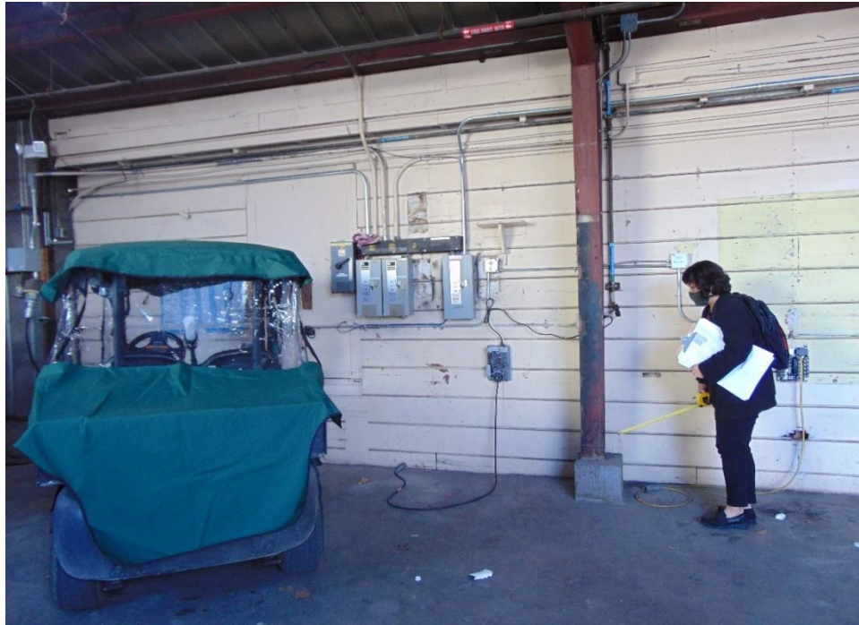
Figure 9. Original exterior channel rustic wood siding visible inside one of the additions.
