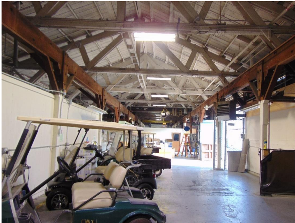
Figure 8. Heavy timber construction and roof trusses inside Building 16.
