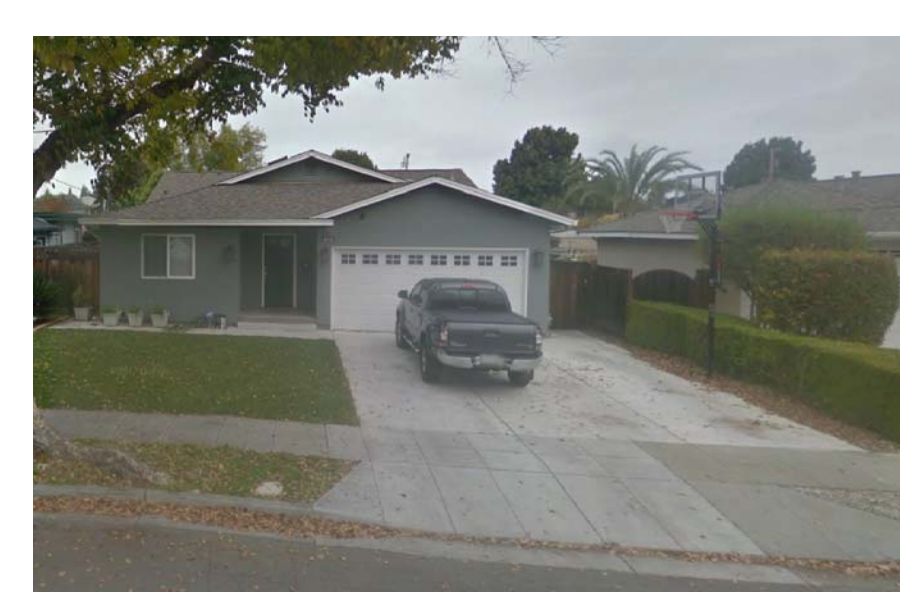
893 LEWIS AVE - FRONT ELEVATION WITH RECESSED ENTRANCE AND FRONT GARAGE - GABLE ROOF FACING THE STREET AND HIP ROOF SLOPING AWAY FROM STREET WITH EXTENSION OVER ENTRY - VENT UNDER THE ROOF PEAK - FRONT YARD WITH PATH CONNECTING TO THE SIDEWALK - PLATE HEIGHT APPROXIMATELY 9'-0" - CALIFORNIA CONTEMPORARY ARCHITECTURE STYLE
