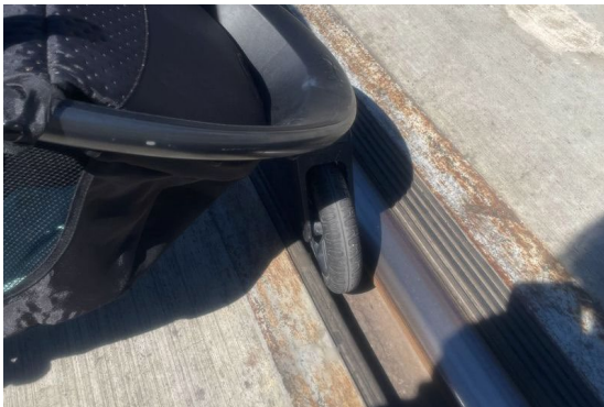
Stroller wheels getting stuck in the tracks at the grade crossings
