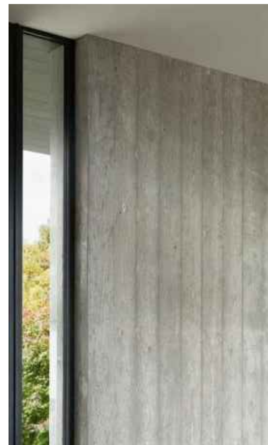
Board-form Concrete (or sim.)
