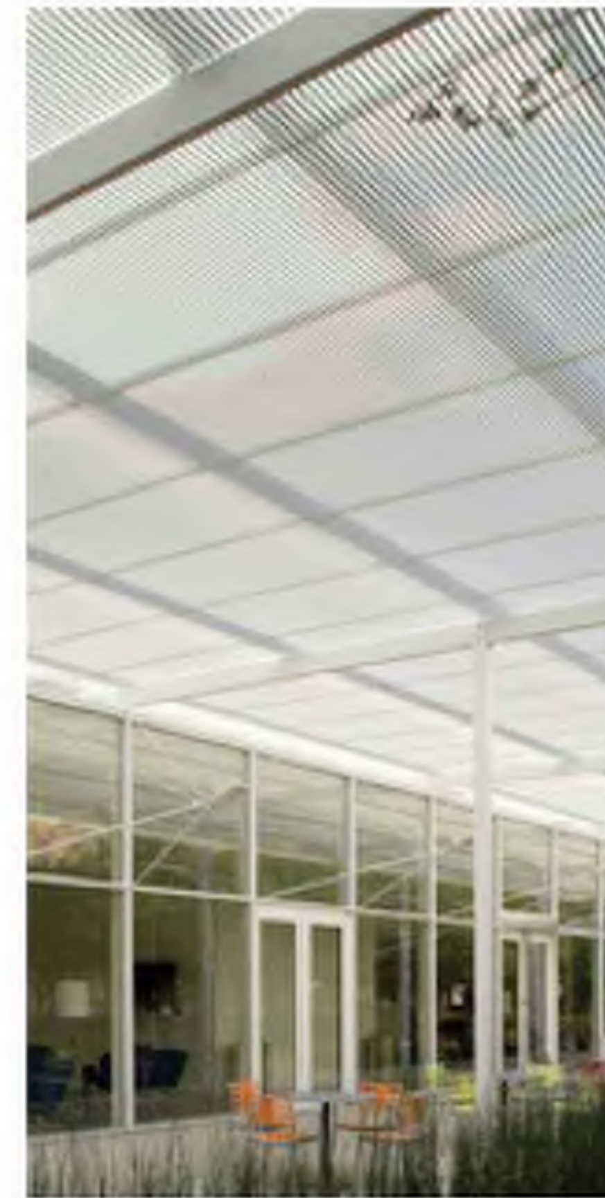
METAL, PAINTED WHITE OFFICE BUILDINGS (MTL-5)
