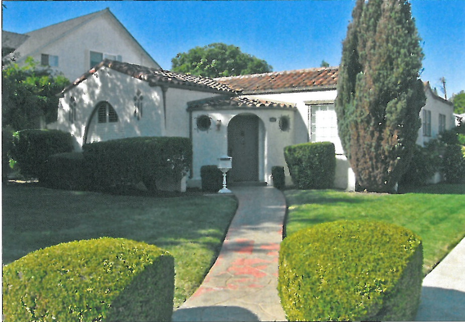
Figure 2. Wesley Davis House, 505 South Frances Avenue.
