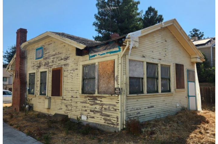
Figure 5: West façade (left) and partial south façade (right), view northeast.
