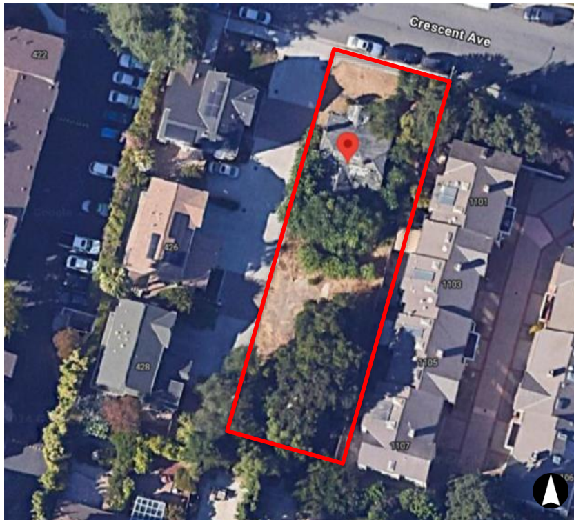
Figure 1: Aerial view 434 Crescent Avenue, the subject parcel outline in red. Source: Google Earth 2024. Edited by Page & Turnbull.
