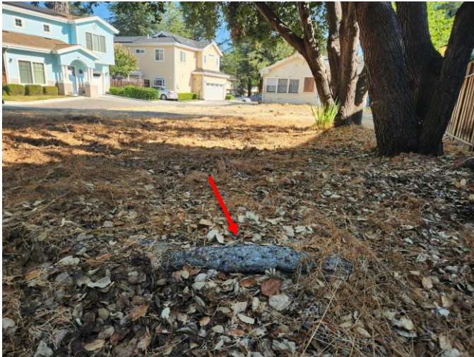
Figure 10: Rear south side of parcel, foundation shown with arrow, view northwest.
