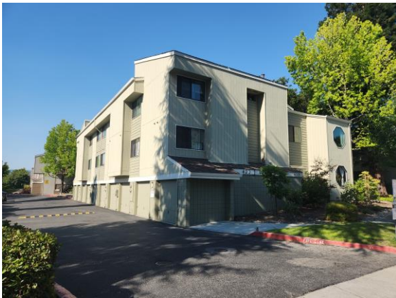
Figure 14: 418-422 Crescent Avenue (built 1982).
