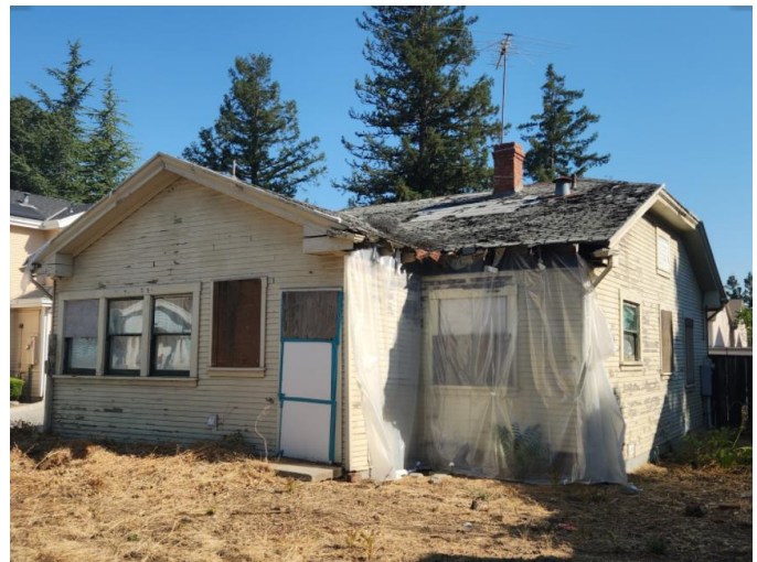
Figure 7: South façade (left) and partial east façade (right), view northwest.
