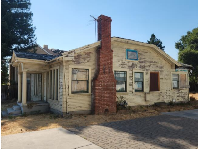
Figure 4: West façade, view southeast.
