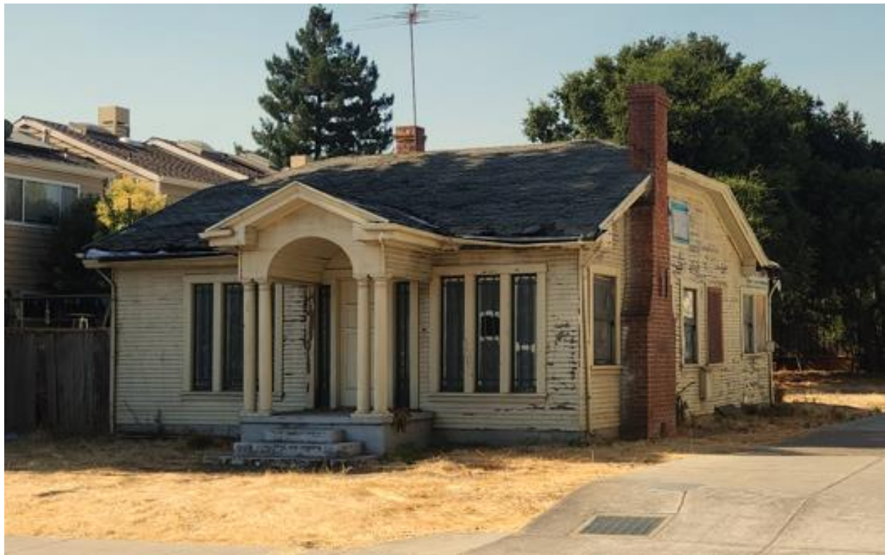
Figure 3: Primary (north) façade of 434 Crescent Avenue, view southeast.
