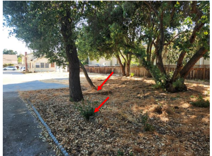
Figure 11: Rear south side of parcel, foundation shown with arrows, view northeast.
