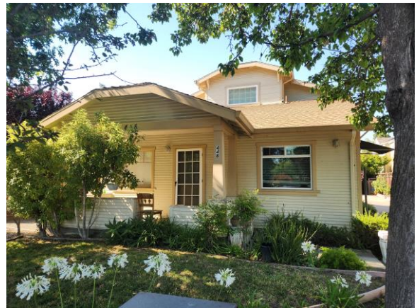
Figure 17: 448 Crescent Avenue (built 1930).
