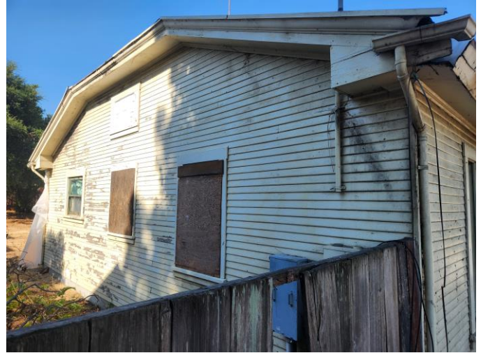
Figure 9: East façade, view southwest.
