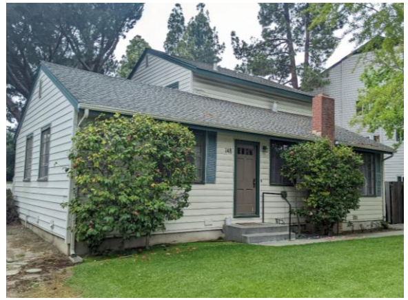
Figure 15: 148 Crescent Avenue (built 1953).
