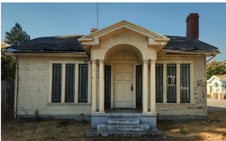
Figure 2. North façade, view south.
