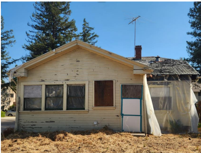
Figure 6: South façade, view north.
