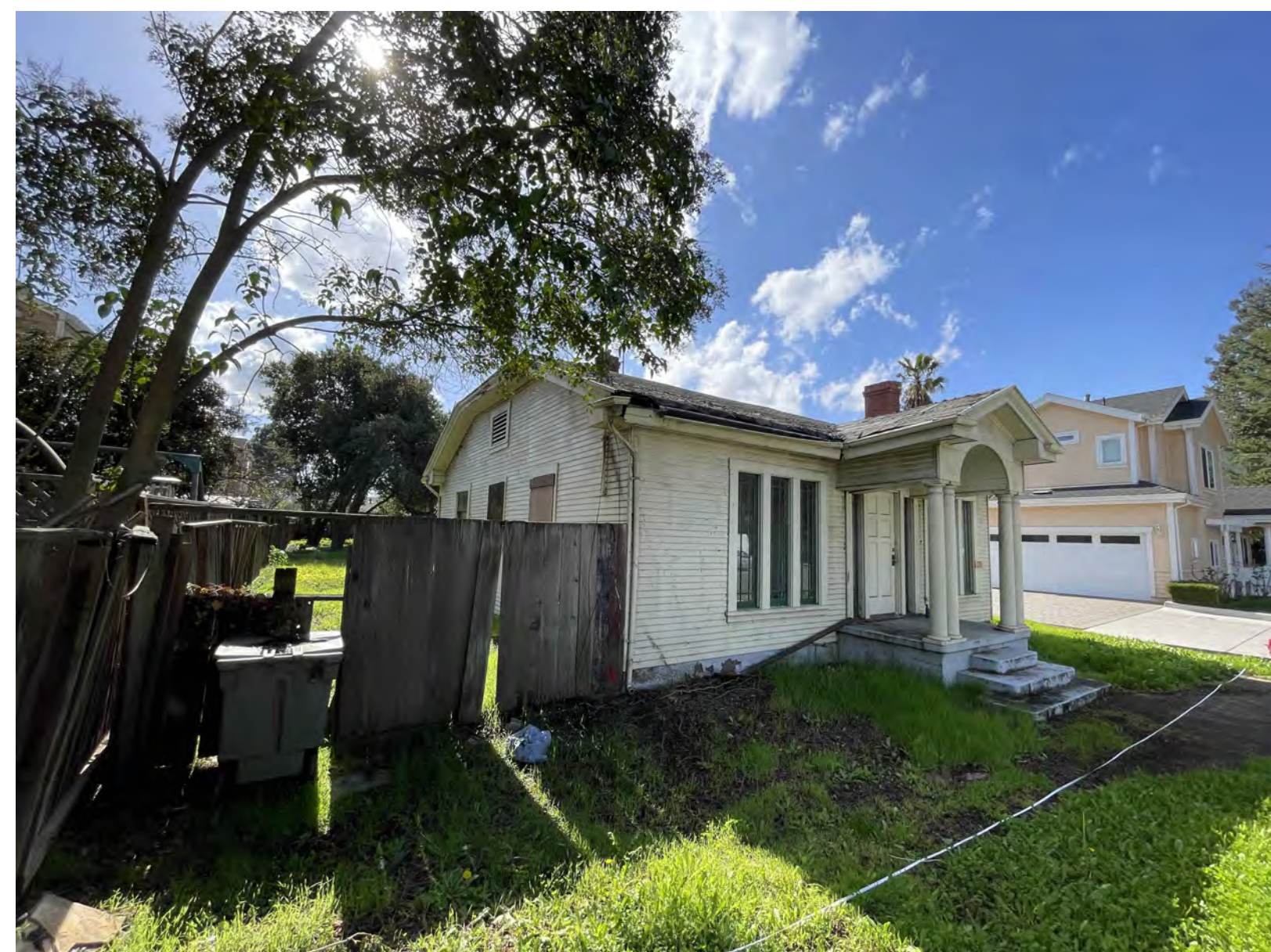
PHOTO #2 - NORTHWEST CORNER
