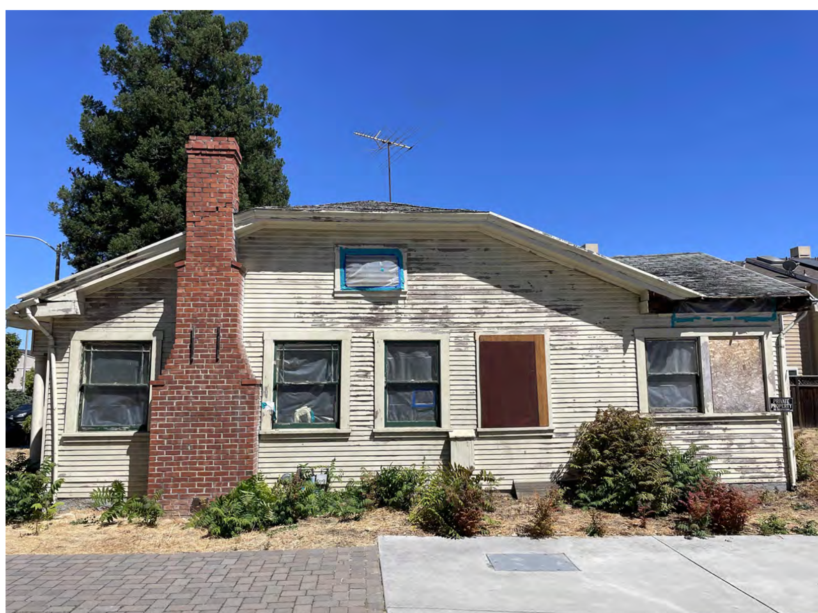
PHOTO #3 - WEST FACADE
