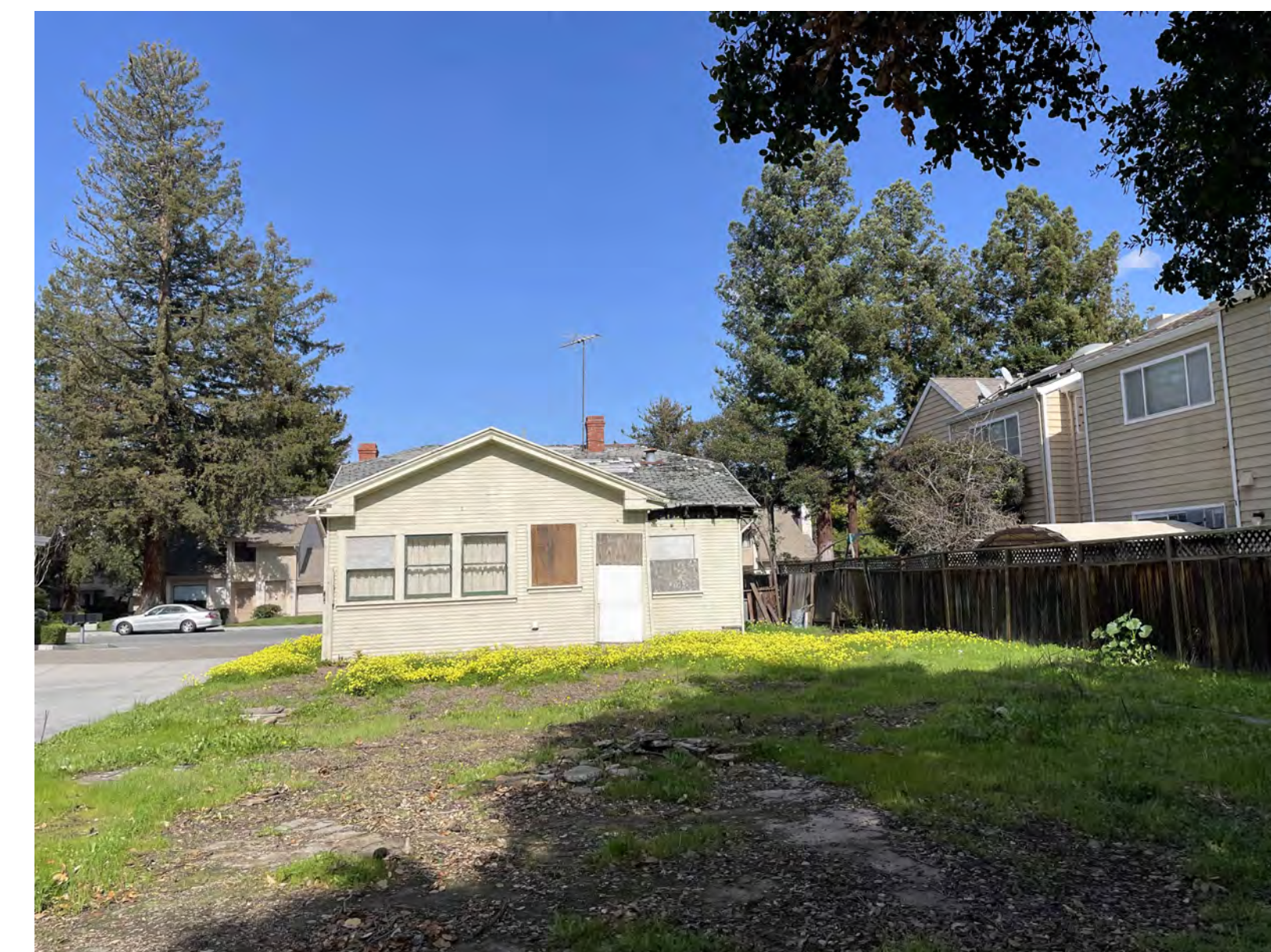
PHOTO #5 - SOUTHERN FACADE
