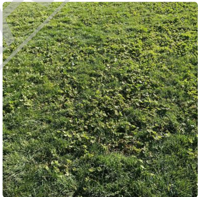
Open turf area, very uneven, many weeds present, clumpy turf. Sunnyvale Middle School Photos
