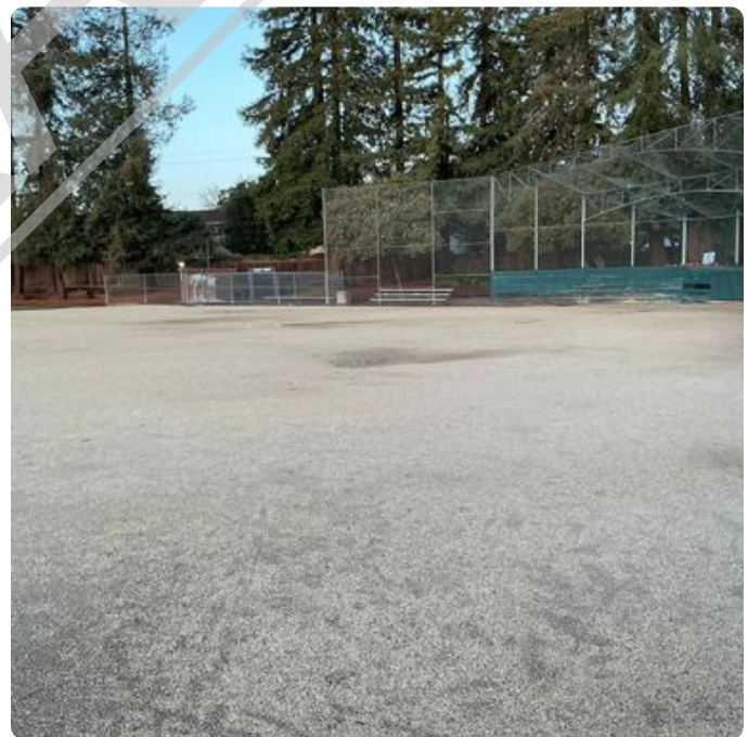
Open turf area, very uneven, many weeds present, bare spots, clumpy turf. Infield edge needs to be manicured and leveled. Las Palmas Park Photos
