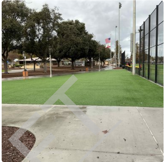
Area outside the field fence containing synthetic turf in good condition. Normally, I would find this area containing bare spots if natural grass. Fair Oaks Park Photos
