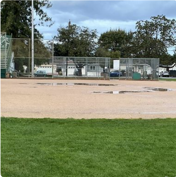
This skinned infield retains water and doesn't drain properly. Washington Park Photos
