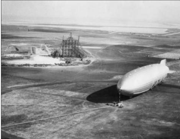
HANGAR 1 IN CONSTRUCTION
