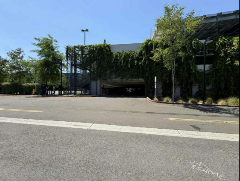
237 MOFFETT PARK DRIVE GARAGE ENTRY SOUTH
