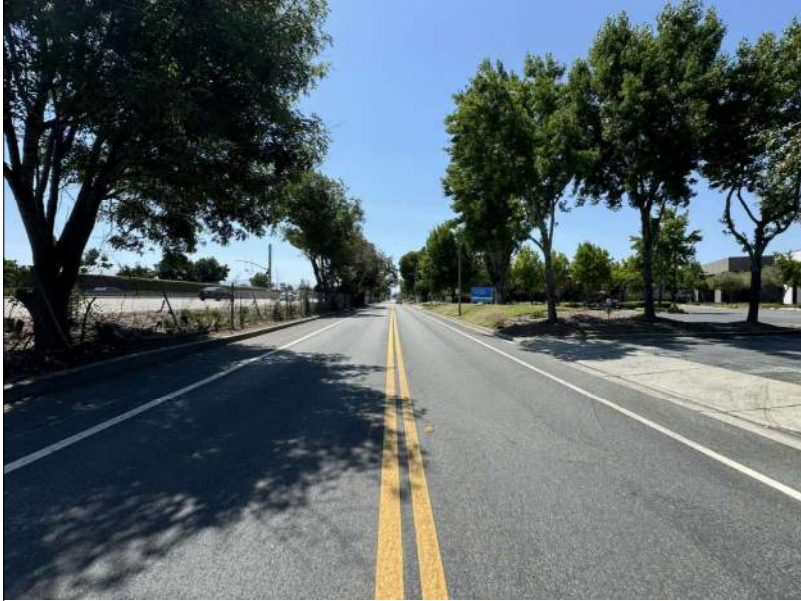
MOFFETT PARK DRIVE EAST LOOKING WEST
