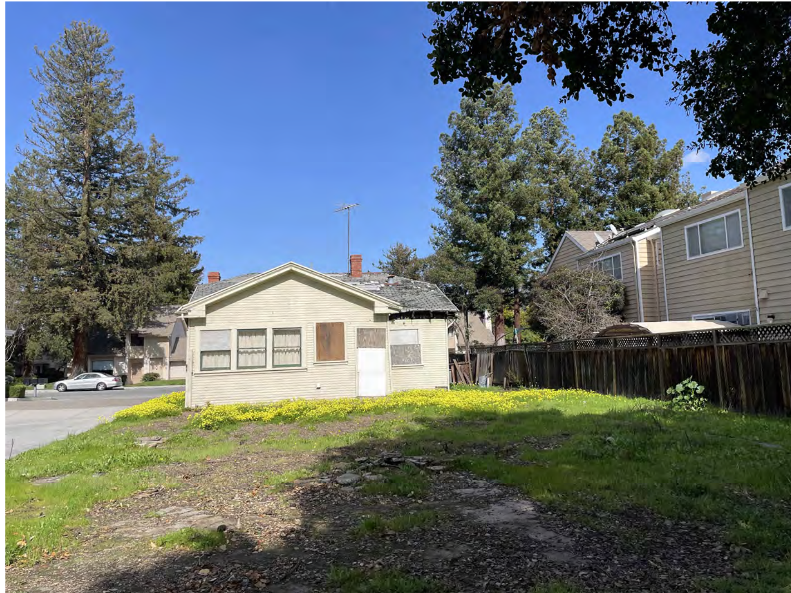
PHOTO #5 - SOUTHERN FACADE
