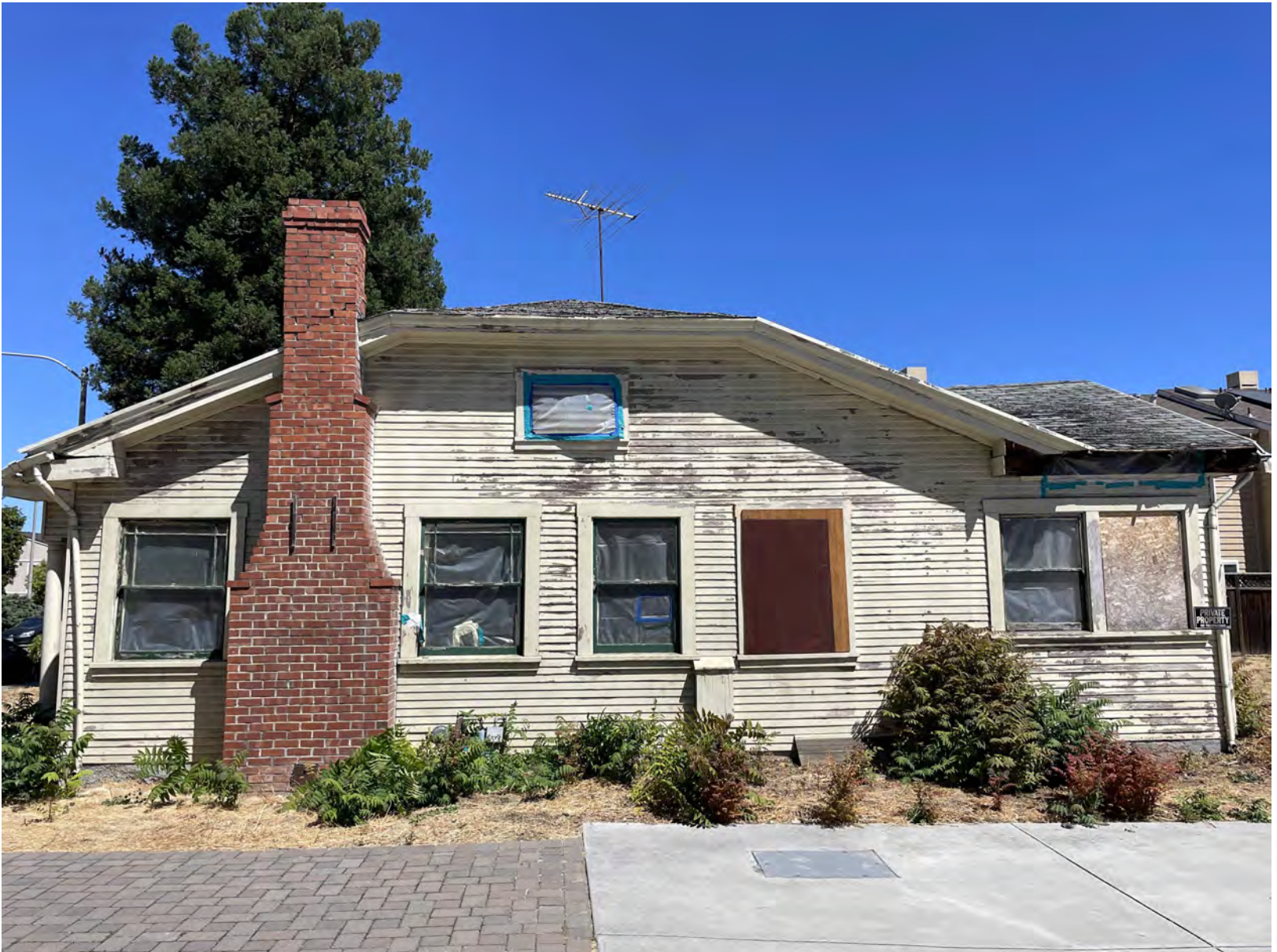
PHOTO #3- WEST FACADE
