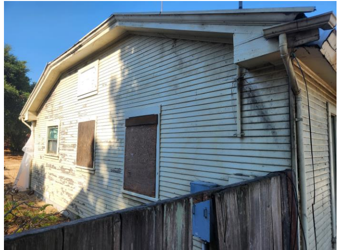
Figure 9: East façade, view southwest.
