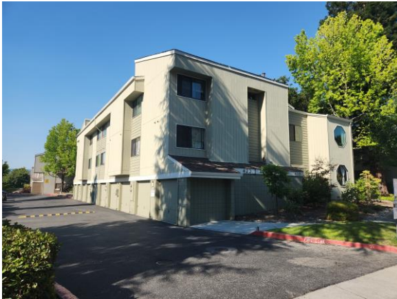
Figure 14: 418-422 Crescent Avenue (built 1982).
