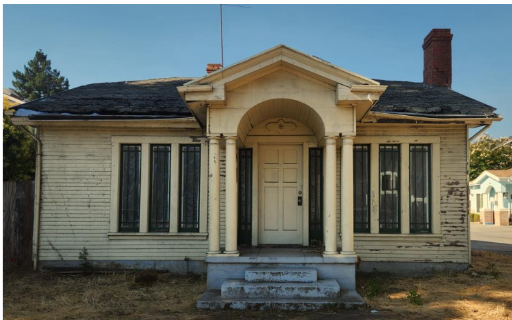
Figure 2. North façade, view south.
