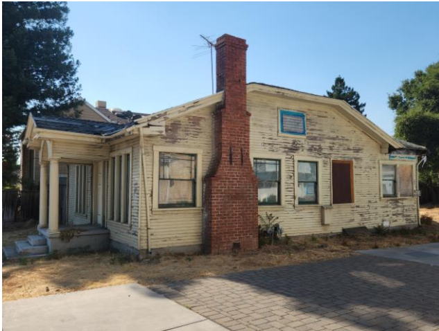
Figure 4: West façade, view southeast.
