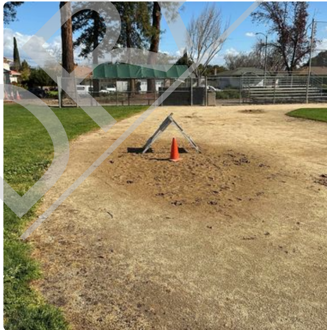
Skinned area exhibits drainage and surface levelling issues. Infield edge needs to be manicured and leveled.
