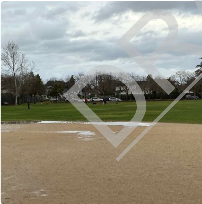
Skinned infield, retains water, doesn't drain properly. Panama Park Photos
