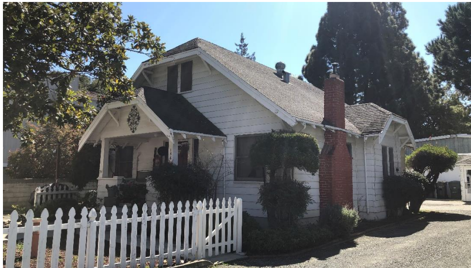
Figure 1. The front (north) and west façades of 156 Crescent Avenue.
