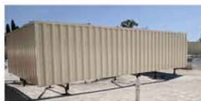
7 R.T.U. SCREEN WALL BEYOND EXAMPLE ONLY, MATERIAL TO MATCH VERTICAL METAL SIDING
