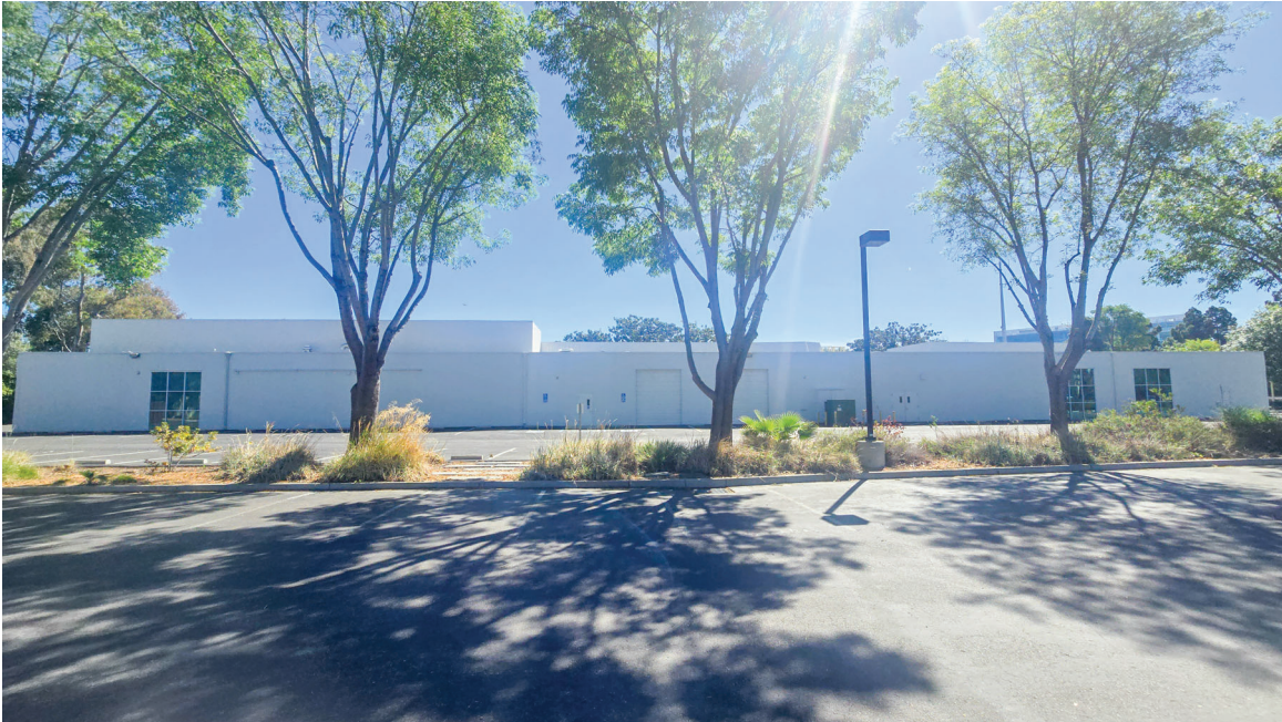
Photo 3: View of 1215 Bordeaux Drive building back facade, facing east from the adjacent parking lot.
