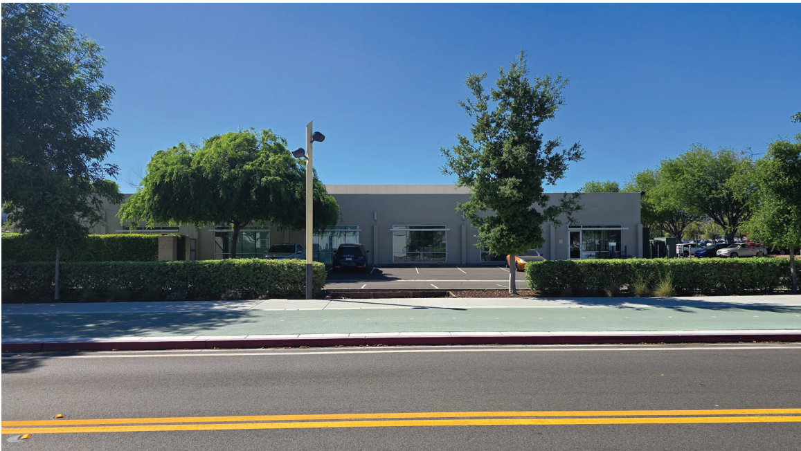
Photo 4: View of adjacent office building across Fifth Avenue, facing south from the project site.
