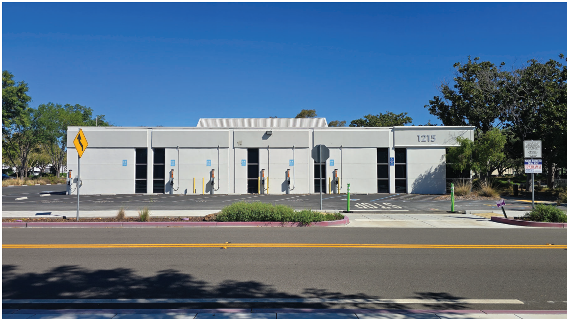
Photo 2: View of 1215 Bordeaux Drive building, facing north from Fifth Avenue.
