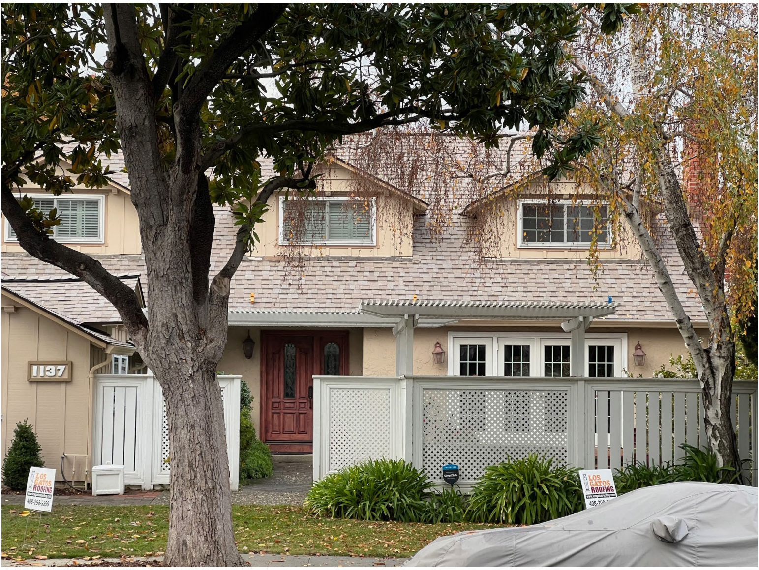
Existing Fence and Arbor Structure (View from the Street) – Built After 1998
