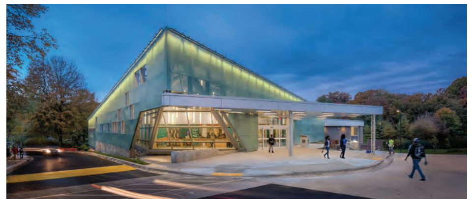
NEW CARROLLTON LIBRARY ADDITION, PROJECT ARCHITECT WITH GWWO INC. New Carrollton, Maryland
