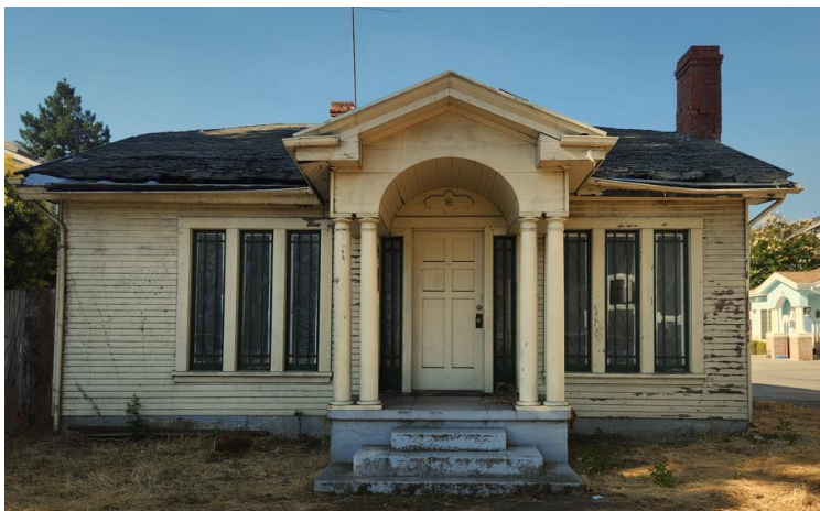
Figure 2. North façade, view south.
