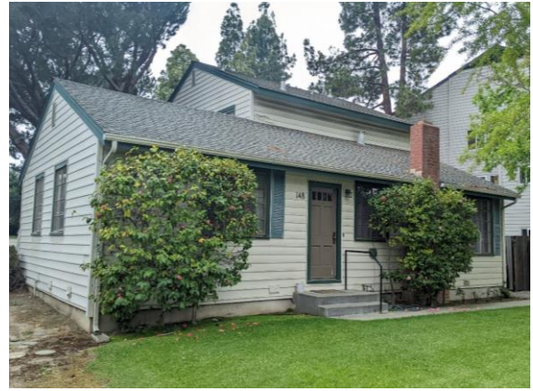
Figure 15: 148 Crescent Avenue (built 1953).
