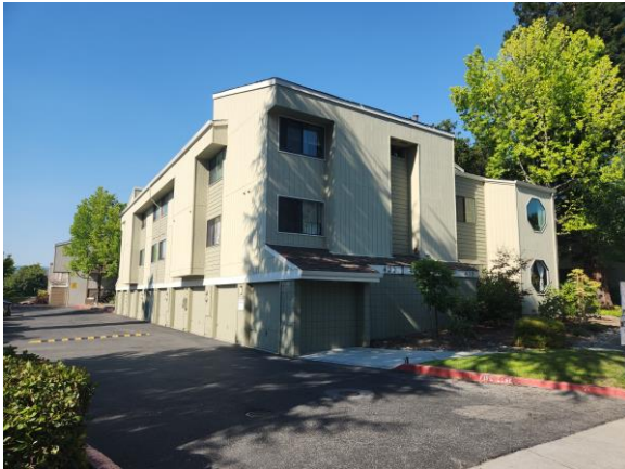
Figure 14: 418-422 Crescent Avenue (built 1982).
