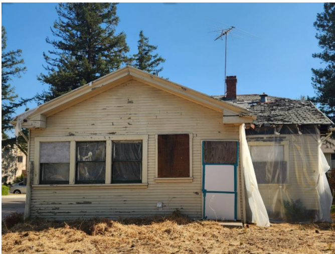
Figure 6: South façade, view north.
