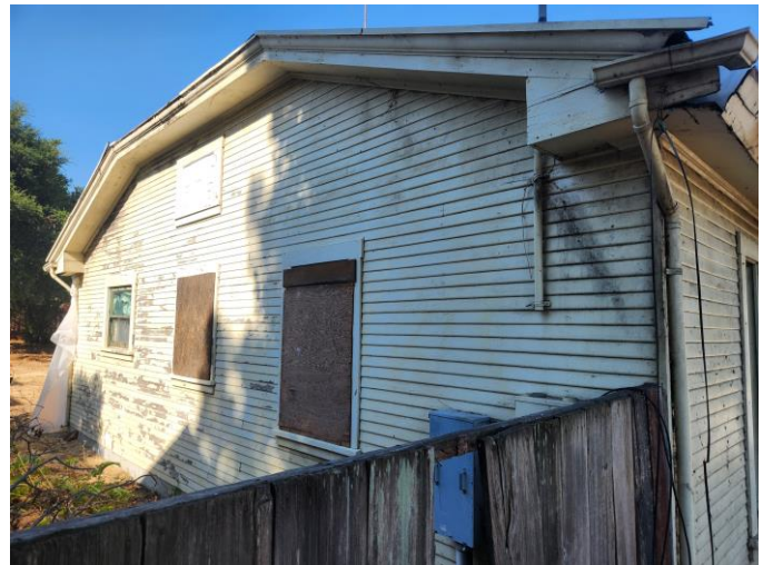
Figure 9: East façade, view southwest.
