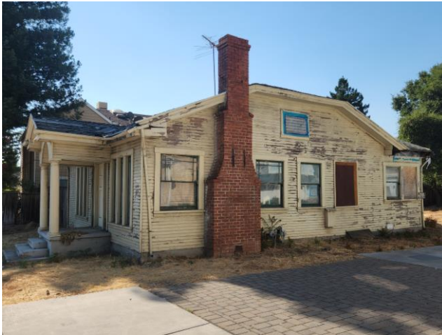
Figure 4: West façade, view southeast.
