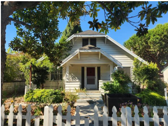
Figure 16: 156 Crescent Avenue (built 1927).
