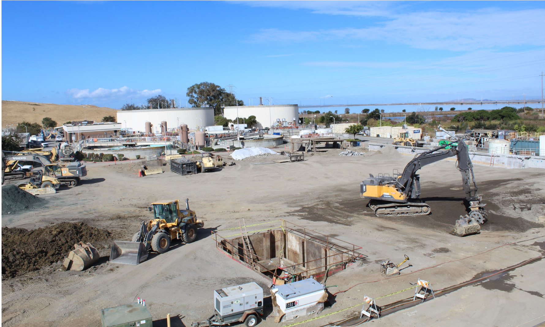
Primary Sedimentation Tank (PST) Demolition
