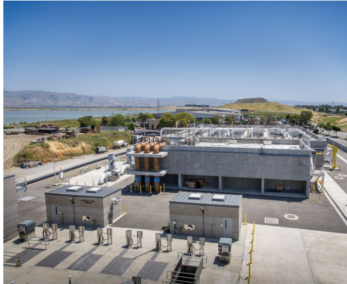
Sunnyvale Water Pollution Control Plant is undergoing a five-phase, 25-year revitalization project that will allow it to accommodate the surrounding region. (Photograph courtesy of Felicia Kieselhorst Photography)
