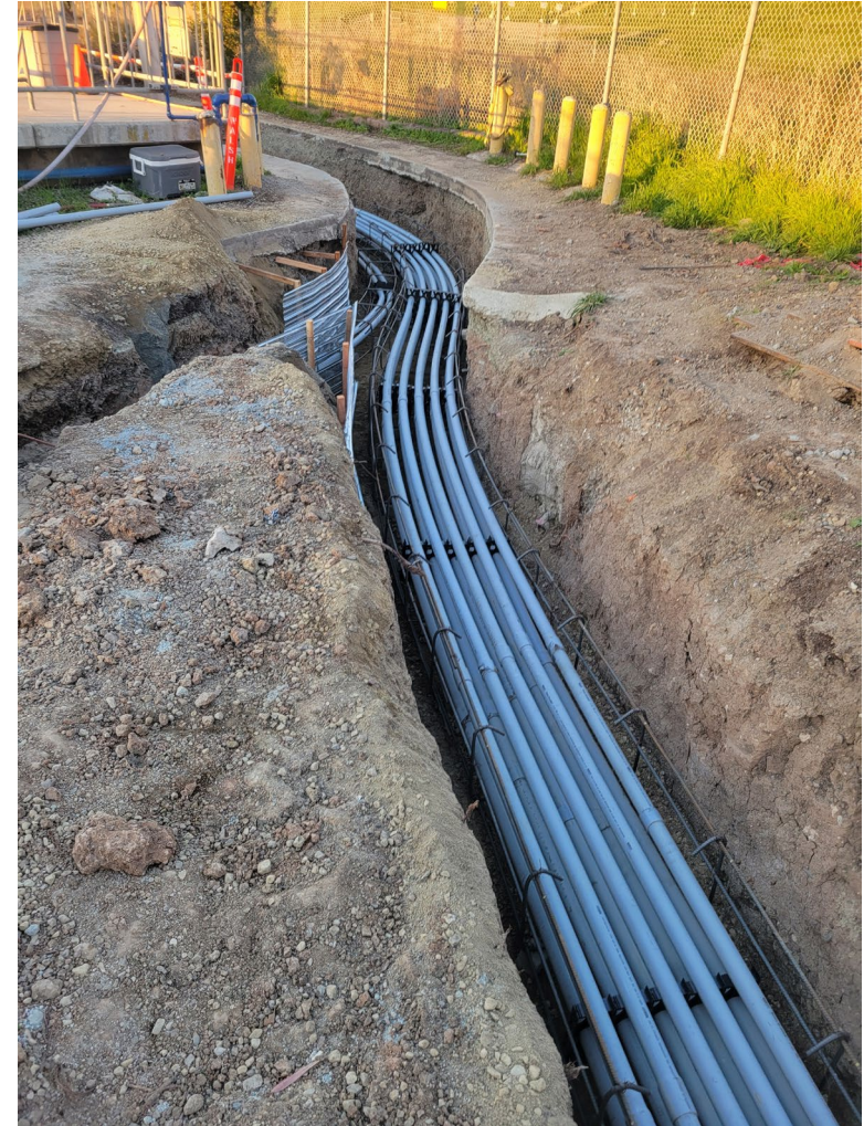
Duct bank installation
