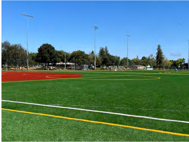
Existing multi-use synthetic turf field with sports field lighting
