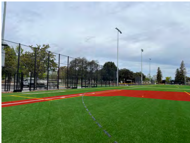
Existing baseball/softball field with sports field lighting
