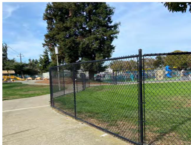
Existing perimeter fencing around field
