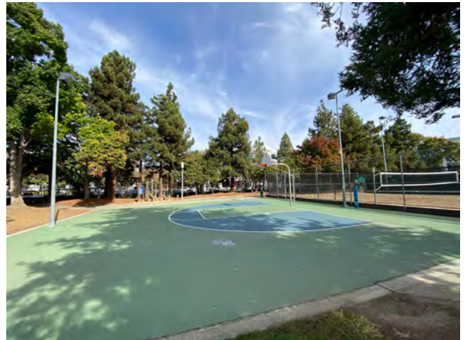
Existing basketball court with court lighting
