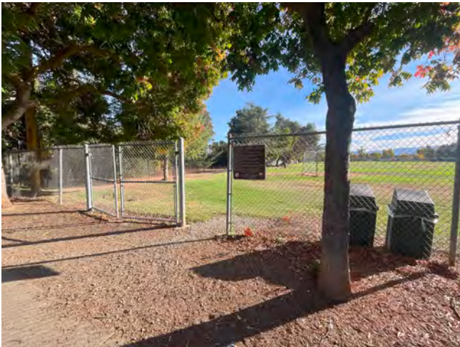
Existing perimeter fence and entrance
