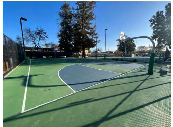
Existing basketball court with court lighting
