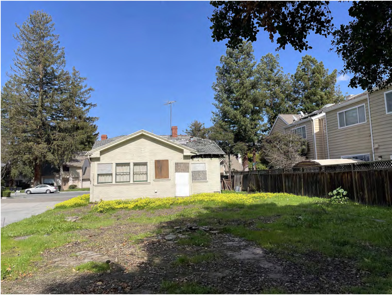
PHOTO #5 - SOUTHERN FACADE
