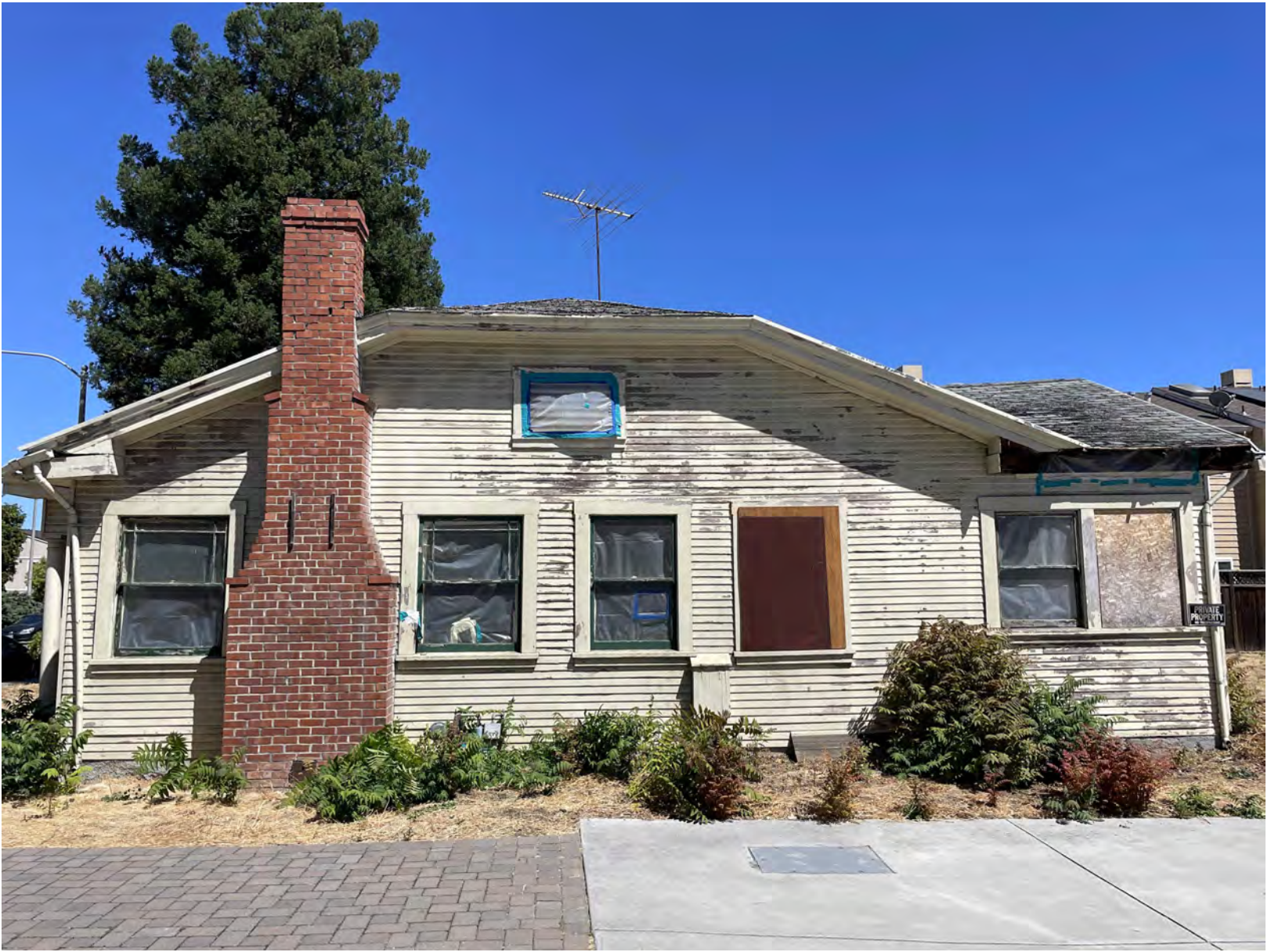
PHOTO #3- WEST FACADE
