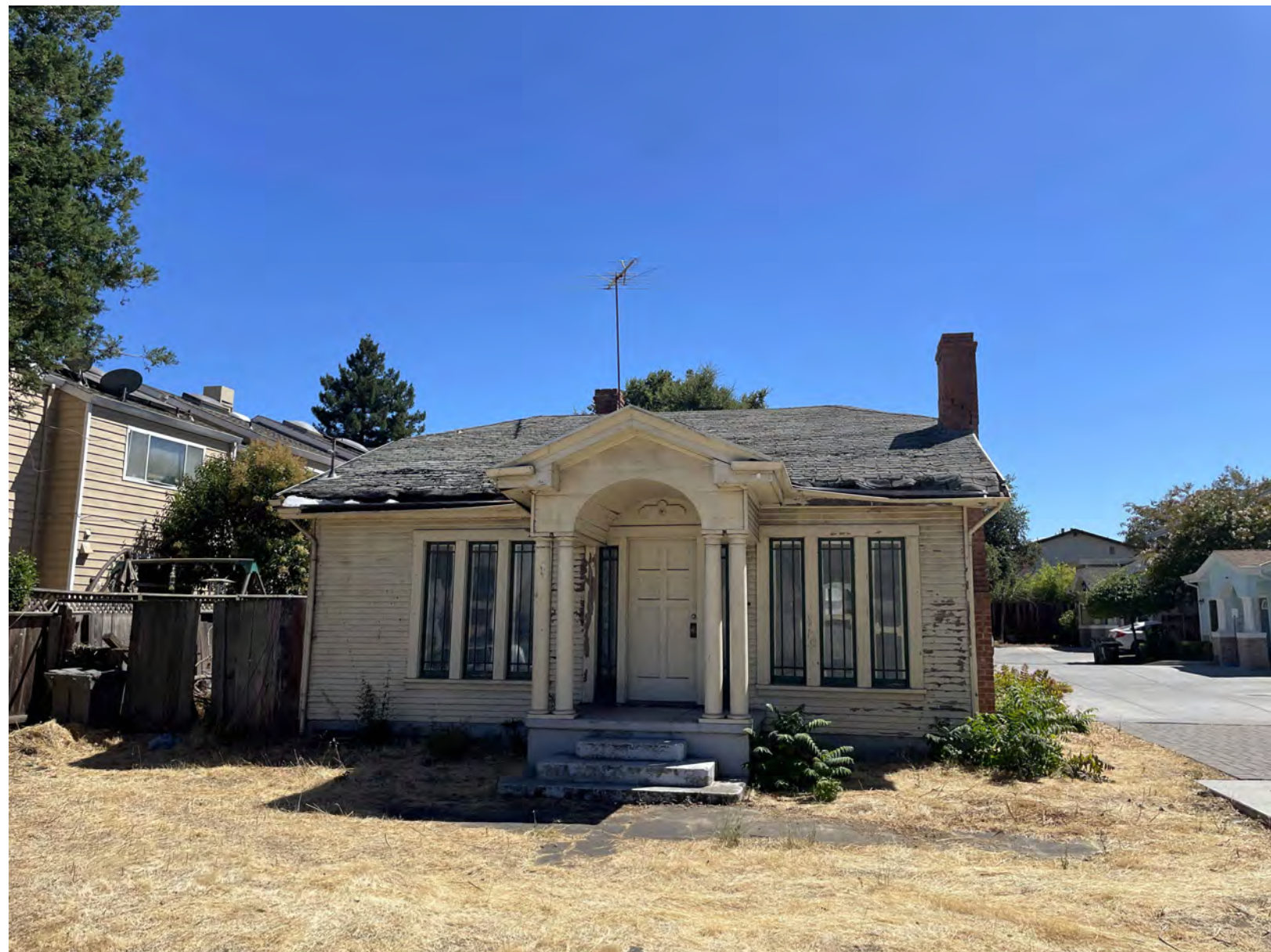
PHOTO #1 - NORTHERN FACADE
