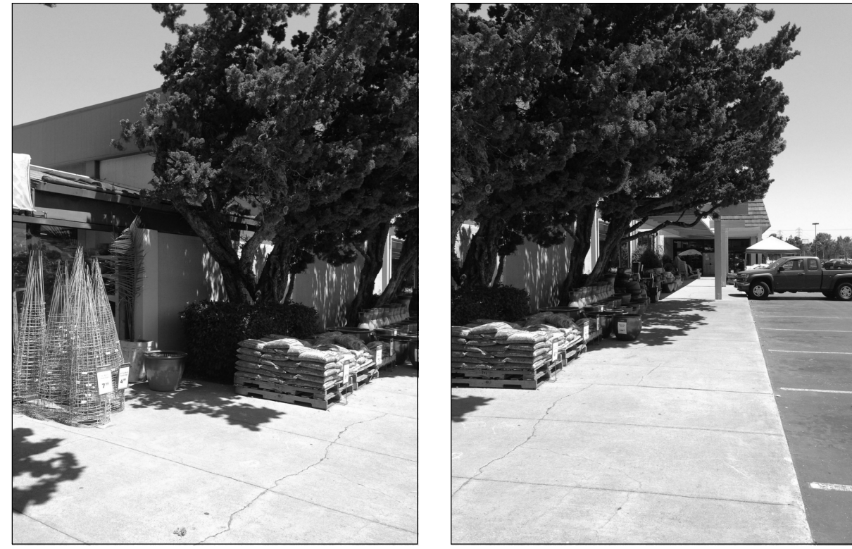
BUILDING SITE PHOTOS N.T.S. (C)
