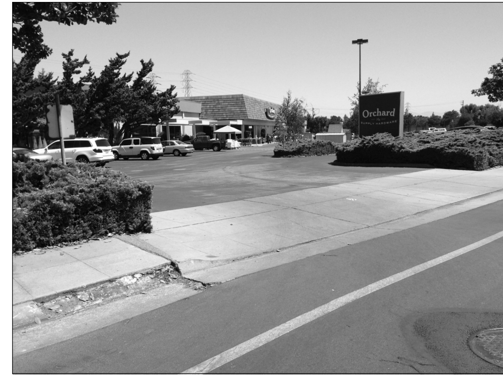
BUILDING SITE PHOTO N.T.S. (B)
