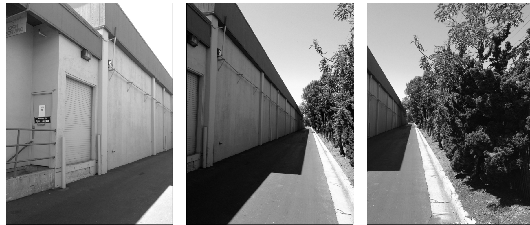
BUILDING SITE PHOTO N.T.S. (I)
