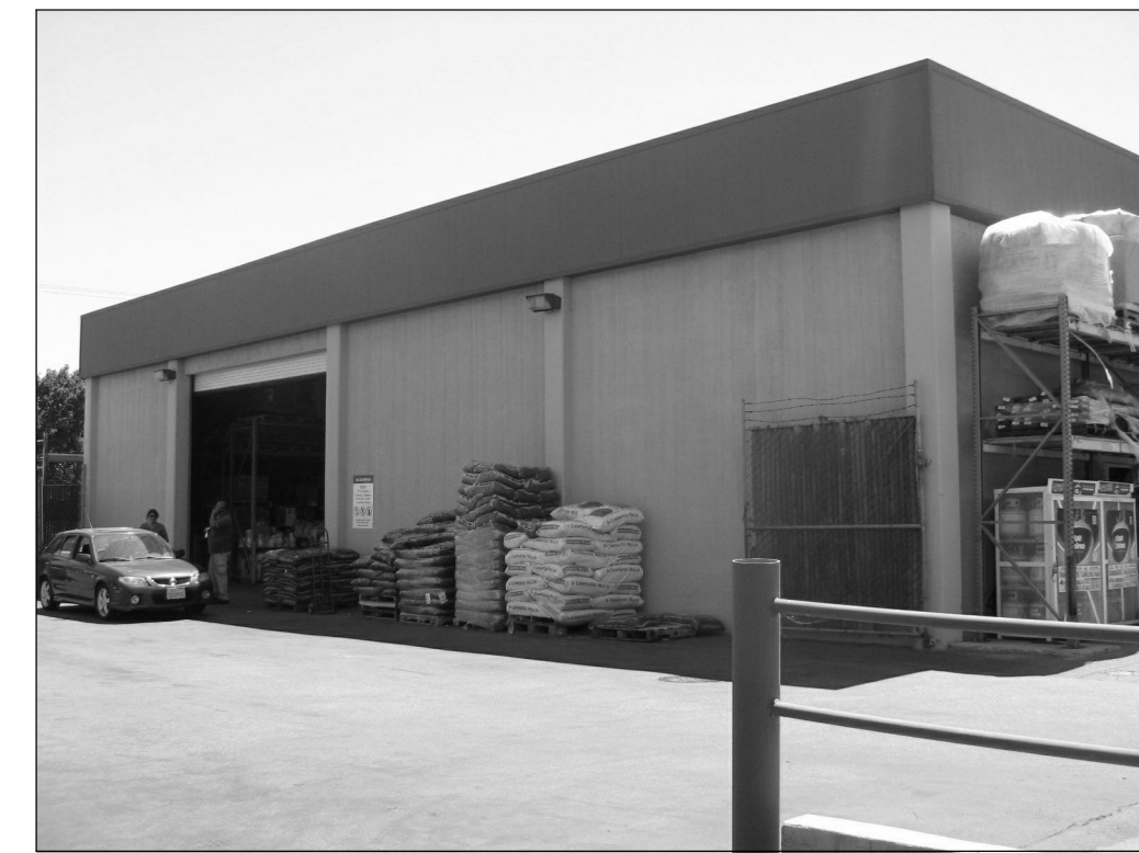
BUILDING SITE PHOTO N.T.S. (G)
