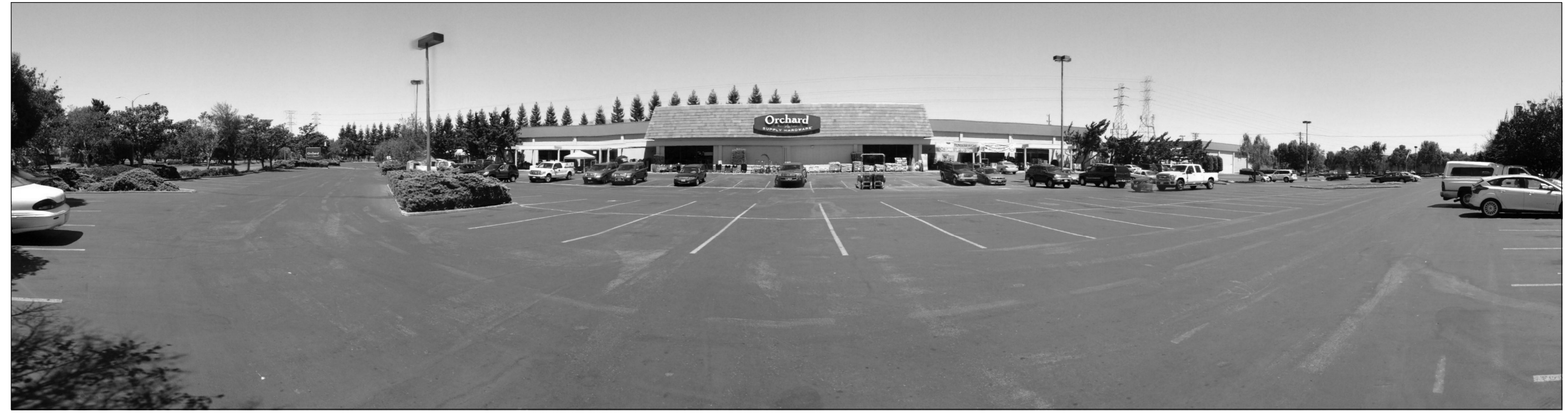
BUILDING SITE PHOTO N.T.S. (A)
