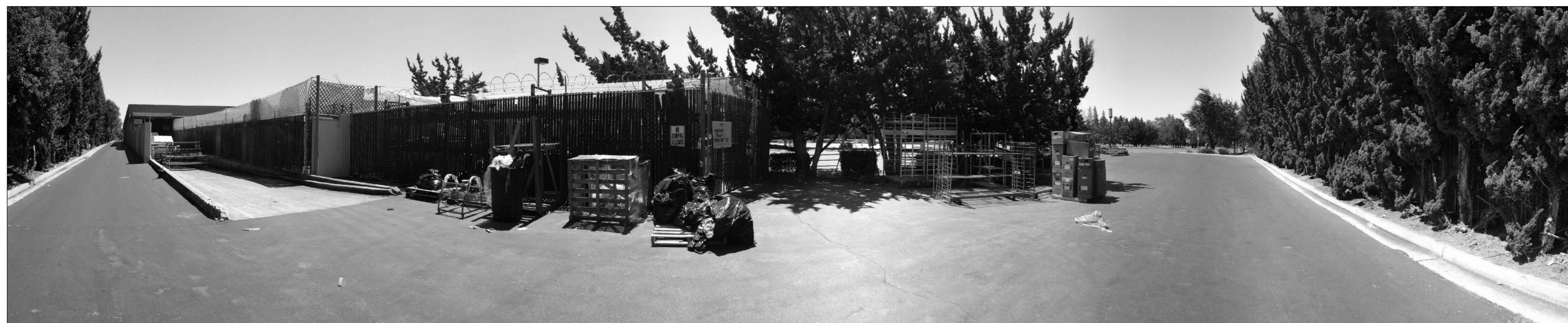
BUILDING SITE PHOTO N.T.S. (J)
