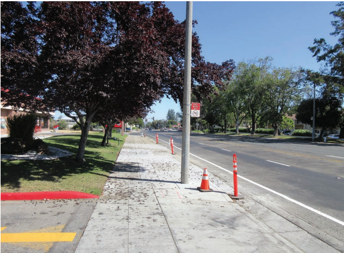
Photo 2: View from the eastern boundary of the project site looking north on South Wolfe Road.
