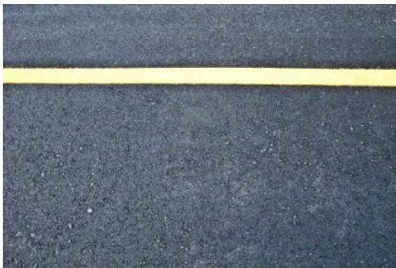
Image 16. Asphalt concrete for access road.
