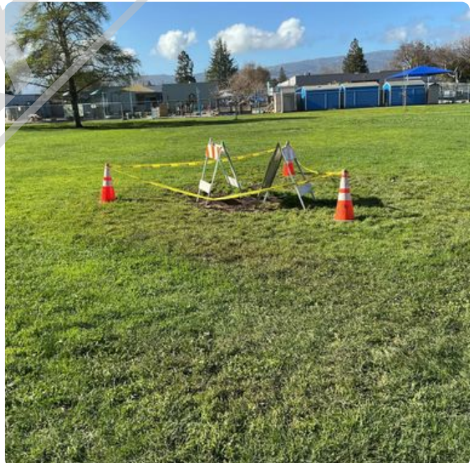
Area of open space that is being repaired. Serra Park Photos
