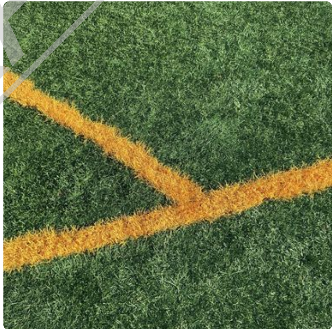
I walked the field, inspecting the seams, the inlaid lines, areas that had evidence of previous repair and I didn't find any area to be unsafe at the time of my observation. Fair Oaks Park Photos
