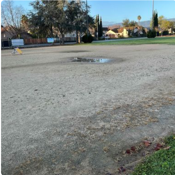
Infield does not drain properly. Ortega Park Photos
