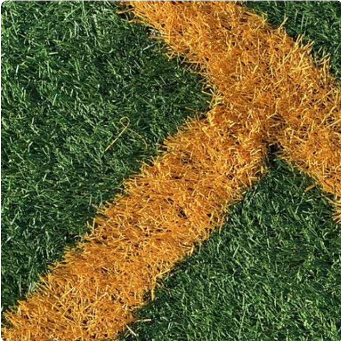
I walked the field, inspecting the areas that had evidence of inlaid lines and I didn't find any area to be unsafe at the time of my observation. Fair Oaks Park Photos
