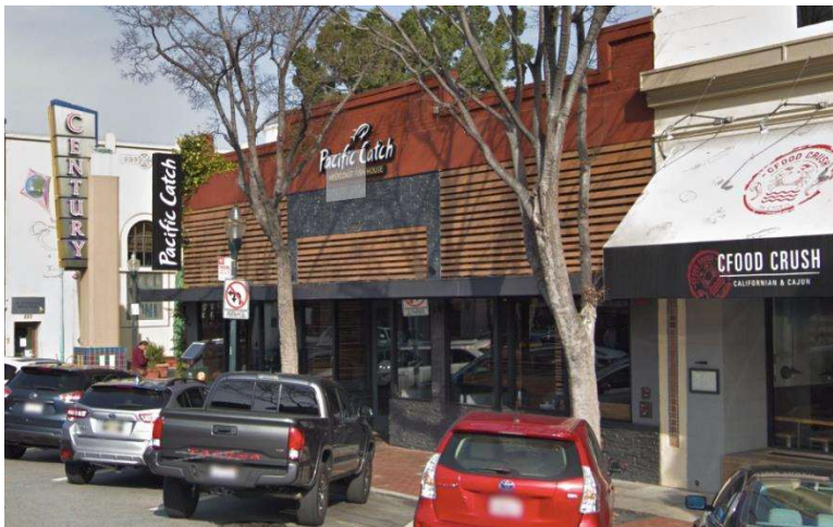
Above: This storefront, in another Peninsula downtown, was recently remodeled. The selection of wood slats for use at the clerestory area reflects the corporate image of this restaurant mini-chain, but does not reflect the traditional material or feature employed at this area of a 1920s-30s storefront.
