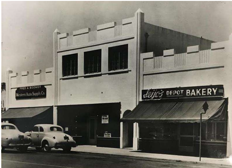
Note the tile work at the storefront base, the stepped parapet, the signage area, and stucco finish at 121-133 S. Murphy Ave.
