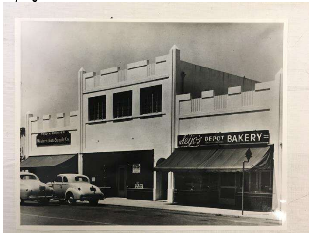
Below: The building just after construction, note no red tile coping at roof line.
