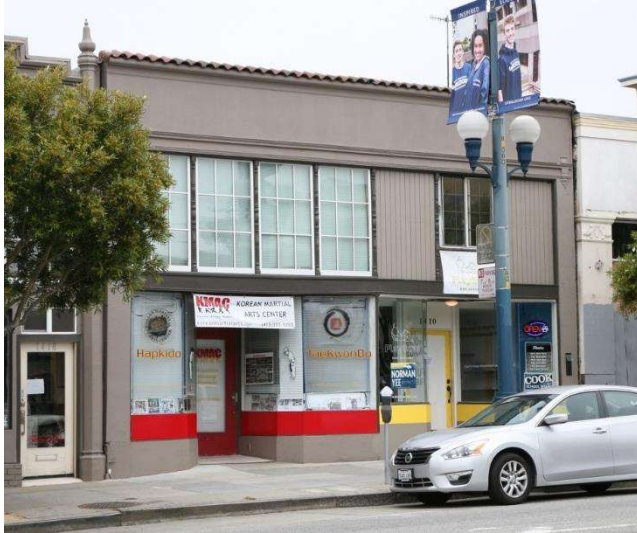
Above: This one-story commercial building has many intact features including its two recessed storefront entries and the detailing enframing the storefront including the large openings for the transom windows. Some transom windows have been lost and the base materials have been changed but the shape, form, massing and major features of this storefront remain.
