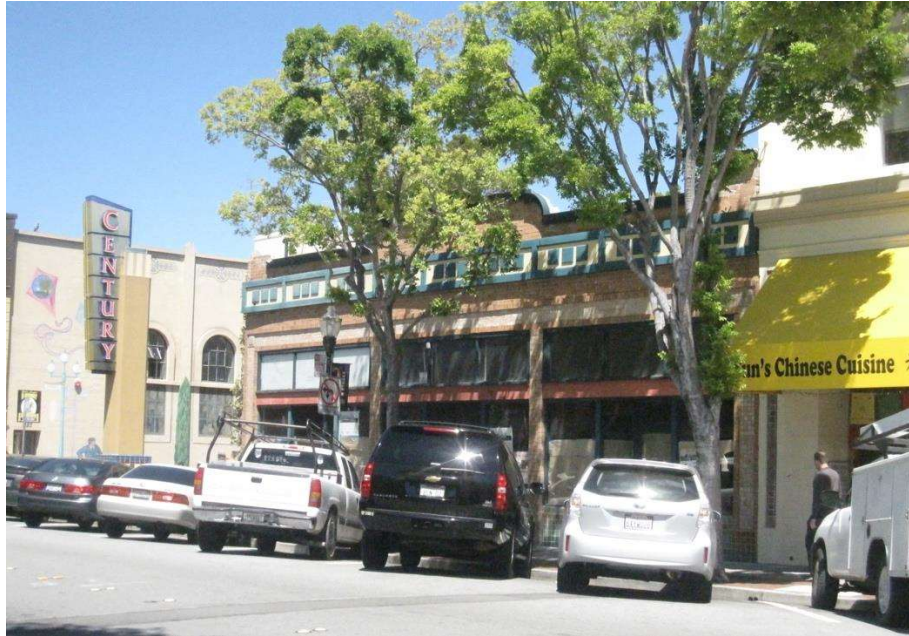
The storefront before it was altered; the clerestory windows were retained behind the wood slats shown above.
