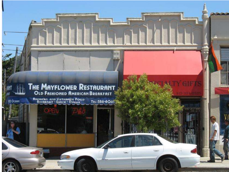
Above: This small-scale, two-storefront corner building would benefit from restoration of the clerestory windows and consistently placed and sized awnings below the clerestory. Varying color of these awnings differentiates the two merchants which can be okay if done well.
