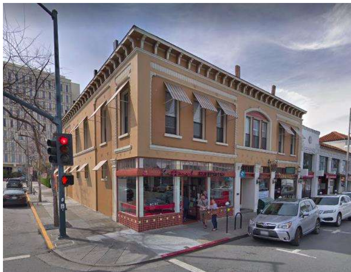
Below: Using awnings at secondary elevations and at second story windows can further highlight the building features, while providing necessary sun shade for building users.
