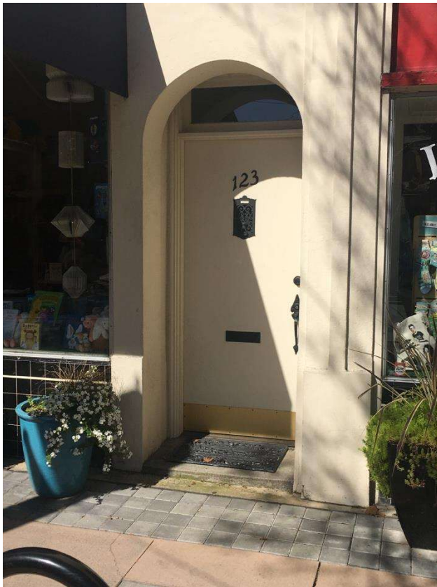
Above: Arched entry to upper story office space.
