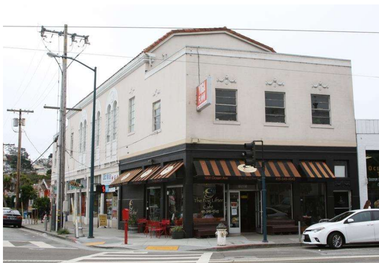
This is a good example of using several awnings of the same size and character along a corner storefront to break up the awning plane and highlight the individual elements of the building.
