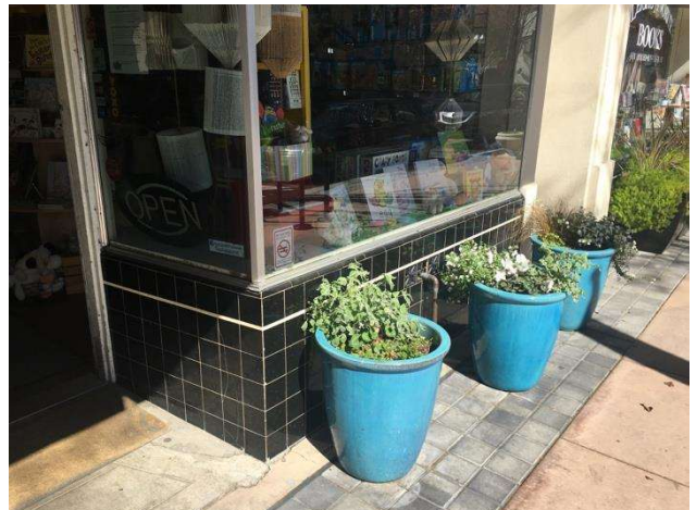
Below: These planters distract from the historic tile at the base of the storefront.
