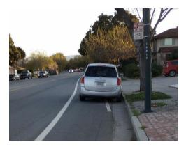
The bike lane clear pavement is reduced to 3' in some segments, which does not meet the VTA BTG guideline of 4'.
