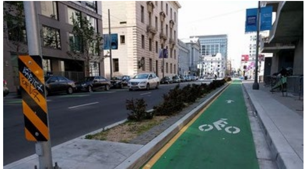
Planted concrete medians
