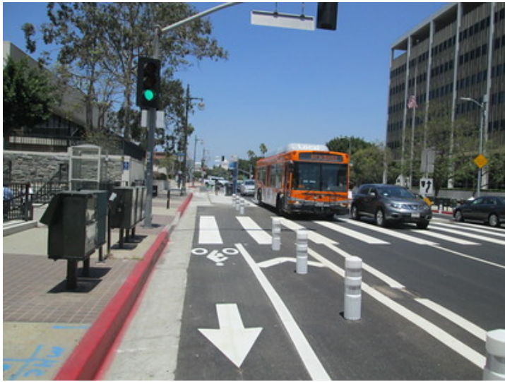
Paint and Flexible Bollards
