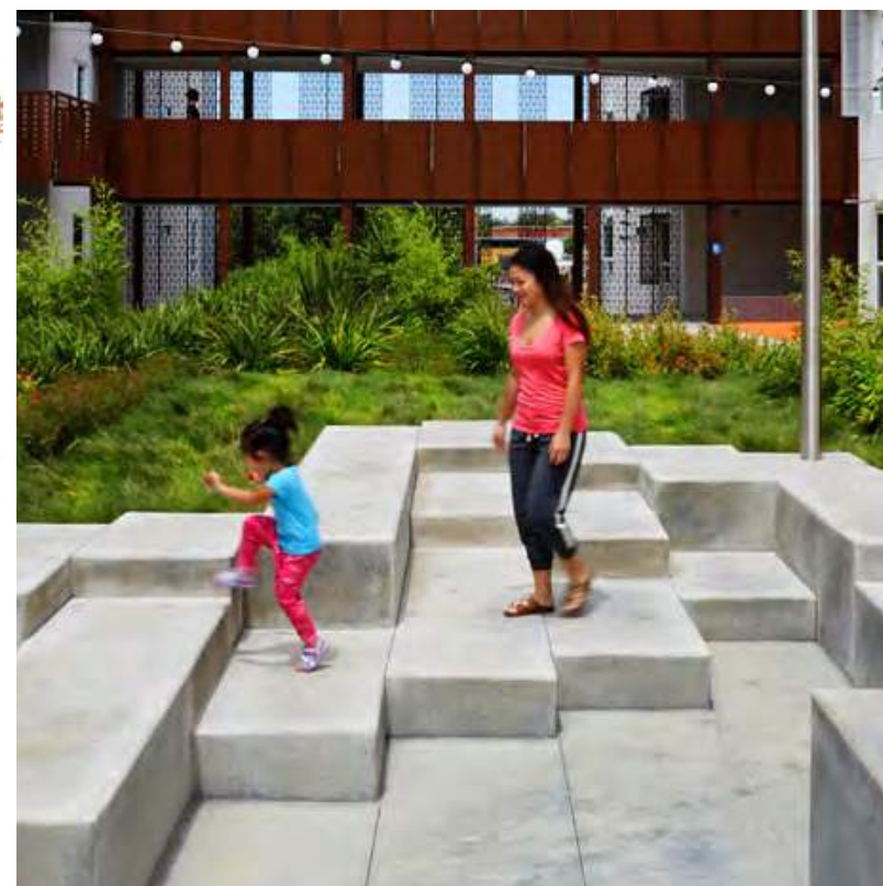
CONCRETE PLANTER - MANUF: DAVIS COLORS - SIZE: LENGTH & WIDTH VARY, HEIGHT 18" - COLOR: PEBBLE
