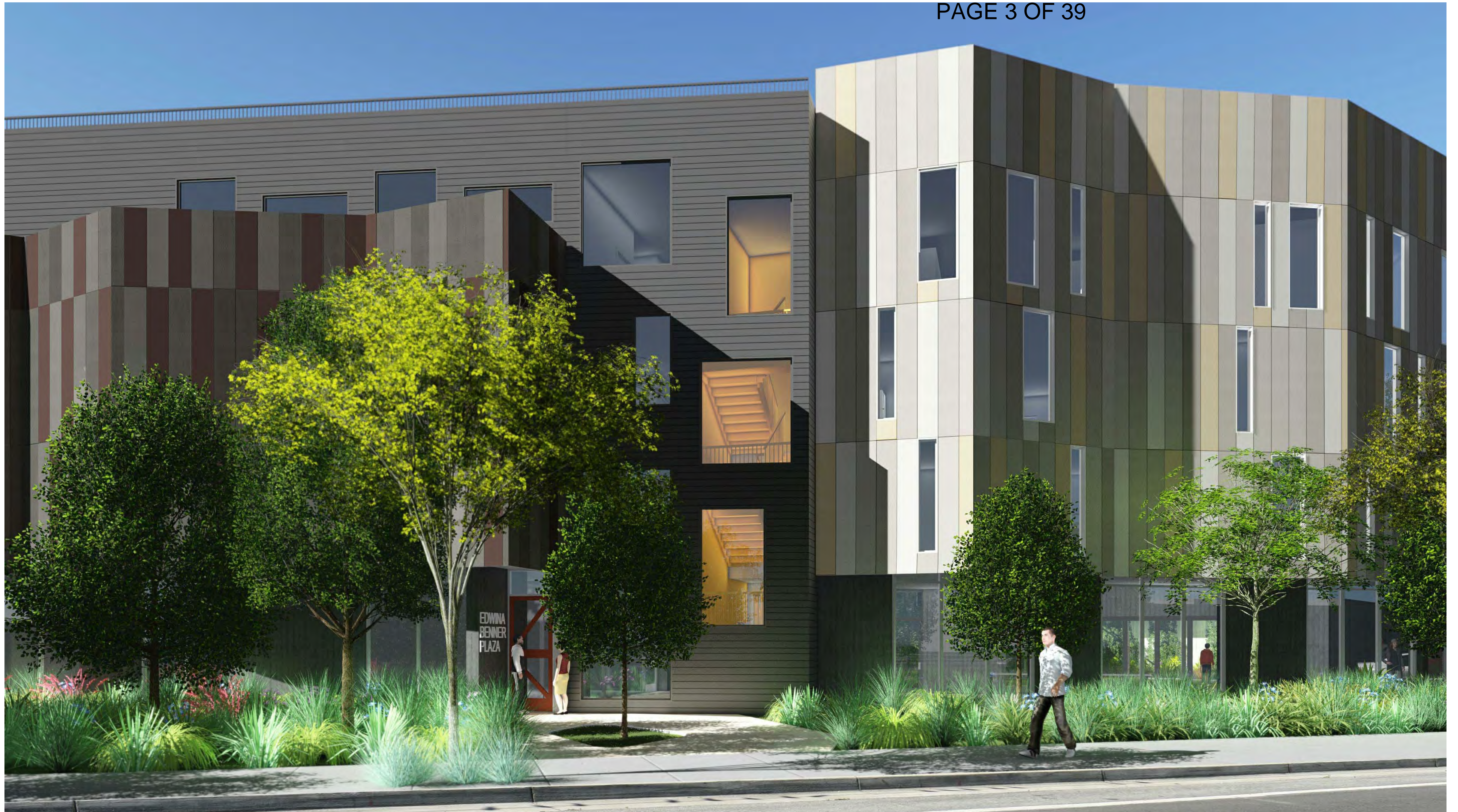
VIEW FROM PERSIAN DRIVE - MAIN ENTRY
