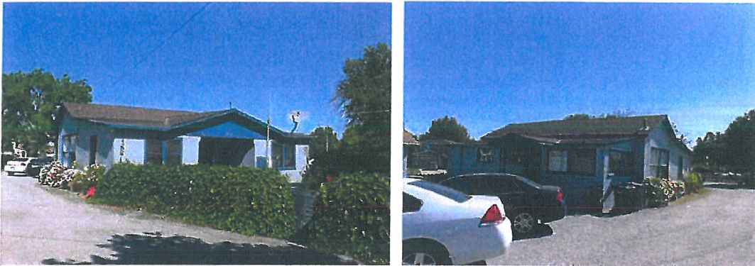
Figures 1 and 2. Dwelling at 1150 Dahlia Court.
