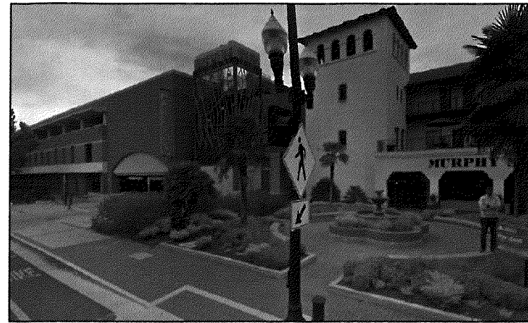
PARKING STRUCTURE + COURTYARD
