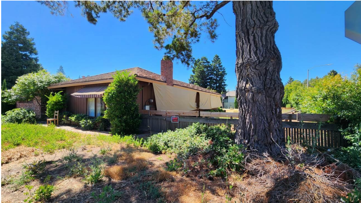
Figure 4: Detail, western facade
