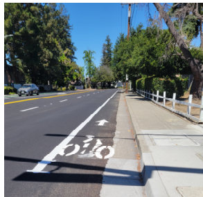
Existing Class II Bike lane on Hollenbeck north of Danforth Dr.
