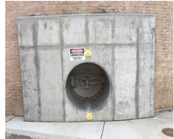
New style side hatch (Digesters 1 and 2)
