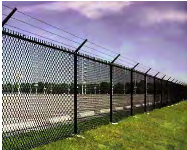
Image 21. Chain-link fence with additional top protection.
