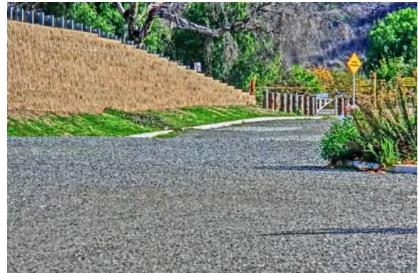
Image 17. Crushed rock surfacing.
