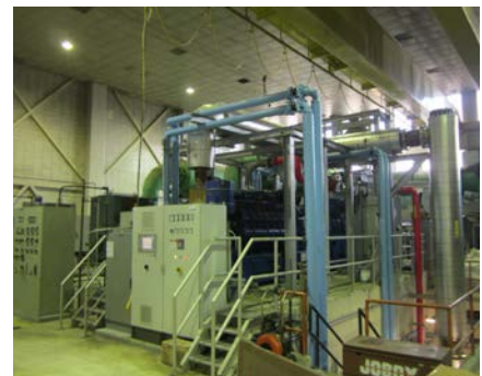
Modern cogeneration engines efficiently convert biogas to heat and power
