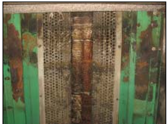
Channel Monster corrosion
