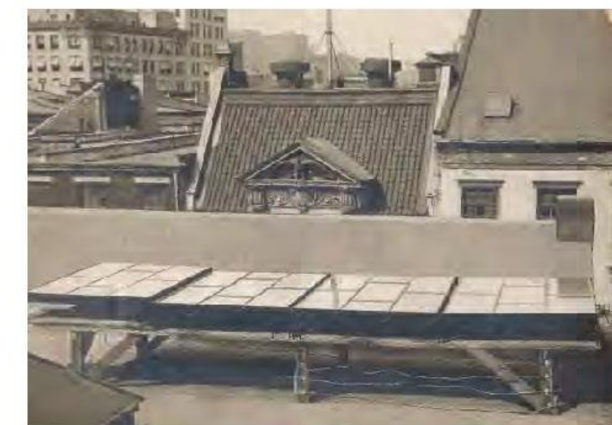
The first solar array installed by Charles Fritts in 1884 in New York City. Fritts built the first solar panels in 1881, reporting that the current was "continuous, constant and of considerable force not only by exposure to
