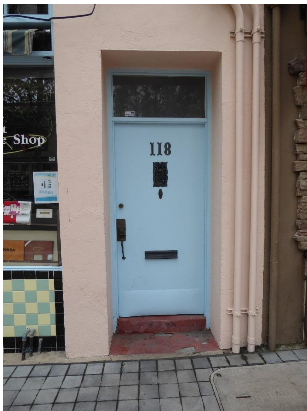
Above: Entry to upper story. Note exposed conduit.
