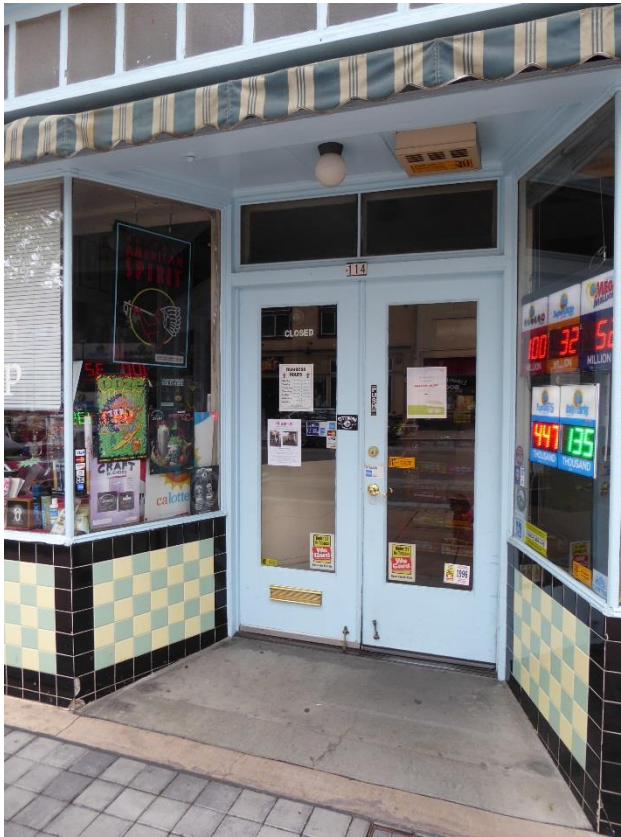
Above: Recessed store entry with original metal storefront windows, multi-colored tile base, and single-panel, glazed, wood double-entry doors with transom above.
