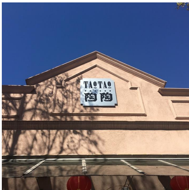
Above: Detail of pedimented false parapet.
