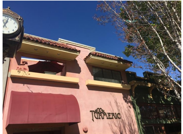
Above: Detail of parapet and fixed and canvas awning.
