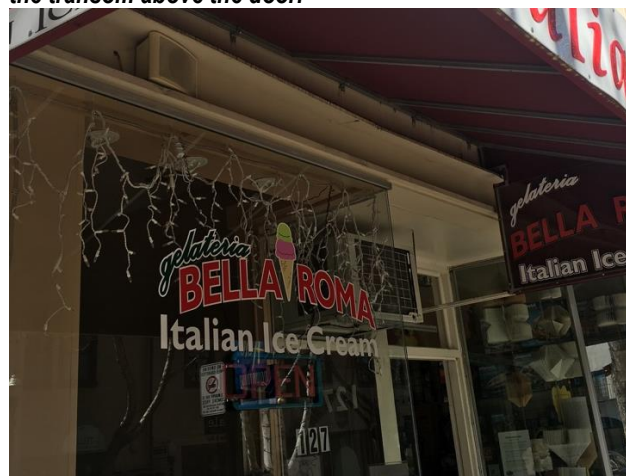
Below: This storefront has a window air conditioning unit in the transom above the door.
