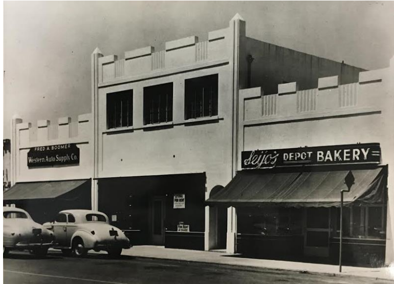
Above: Note the tile work at the storefront base, the stepped parapet, the signage area, and stucco finish at 121-133 S. Murphy Ave.
