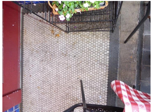
Above: Detail of hexagonal tile entry flooring.
