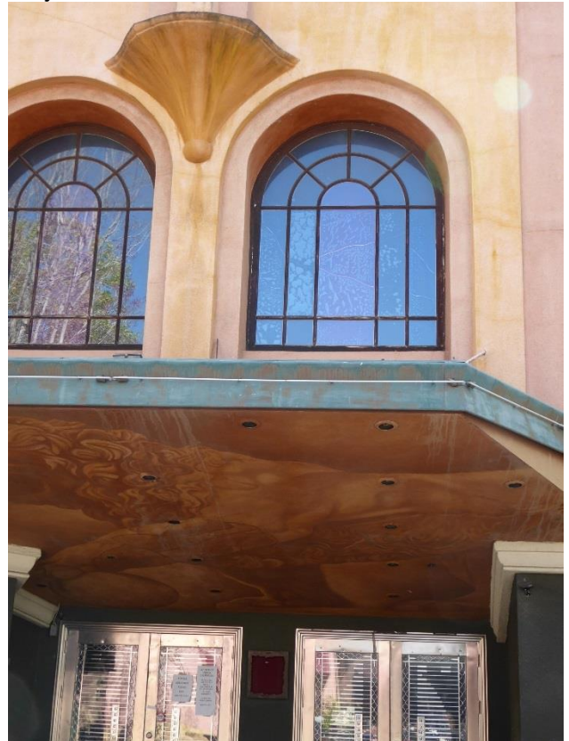
Below: Detail of multi-paned, arched, wood windows above entry
