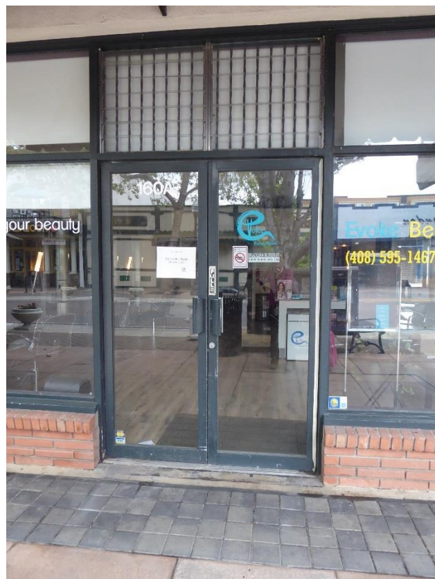
Above: Brick base, wood storefront windows and location of entry doors.
