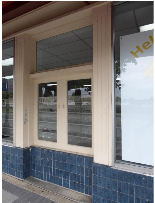
Above: Detail of recessed area, tile base, and fluted wood columns.
