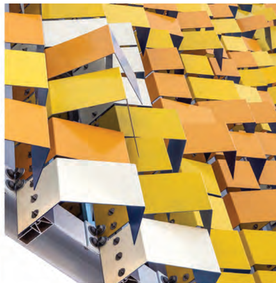
Images above and to the left - Past projects by Artist showing combination of painted aluminum plate elements, fastened to aluminum extrusion structure.
