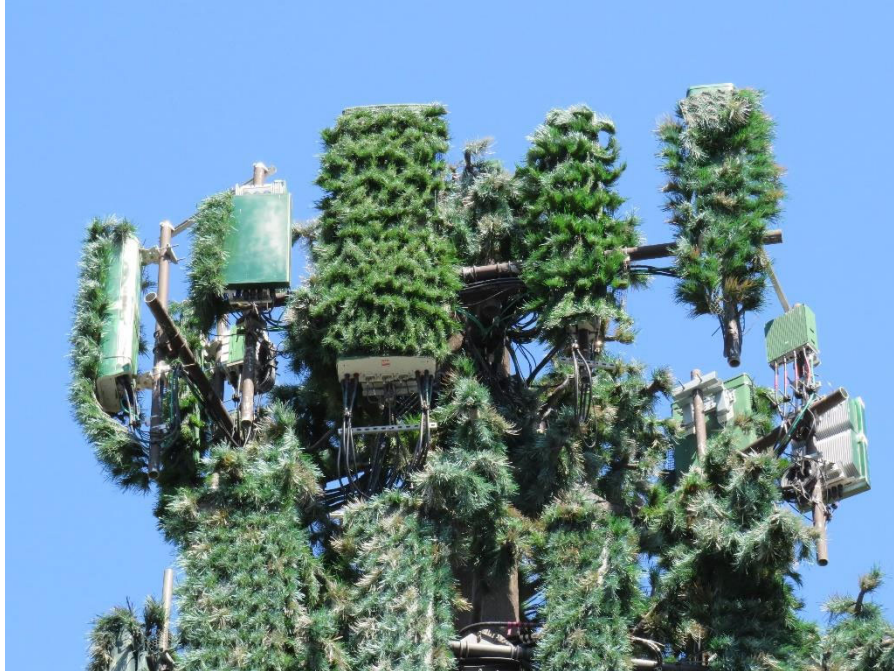
T-Mobile Gamma Sector Antennas #3 (Front)
