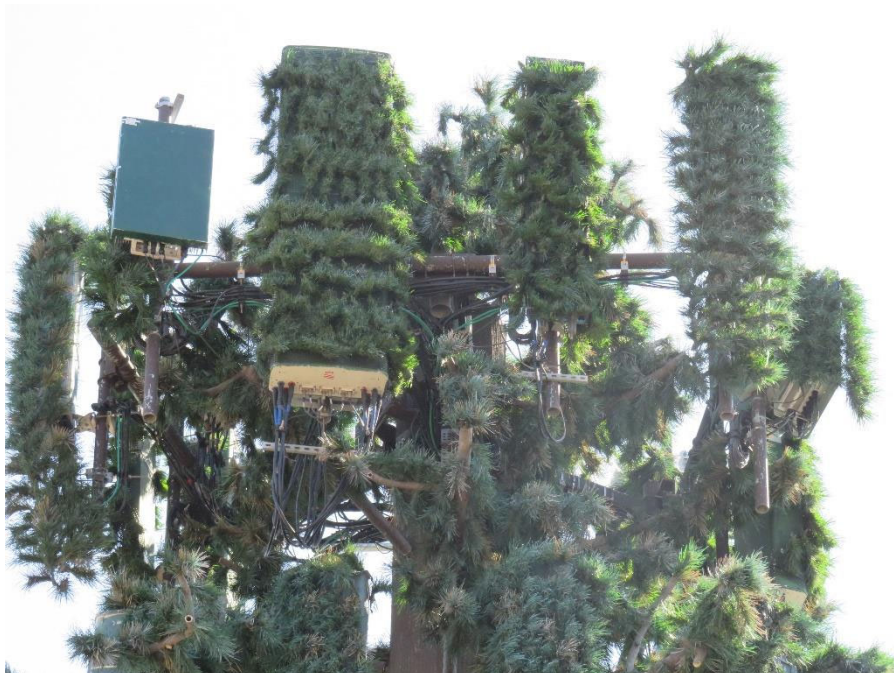
T-Mobile Beta Sector Antennas #2 (Front)
