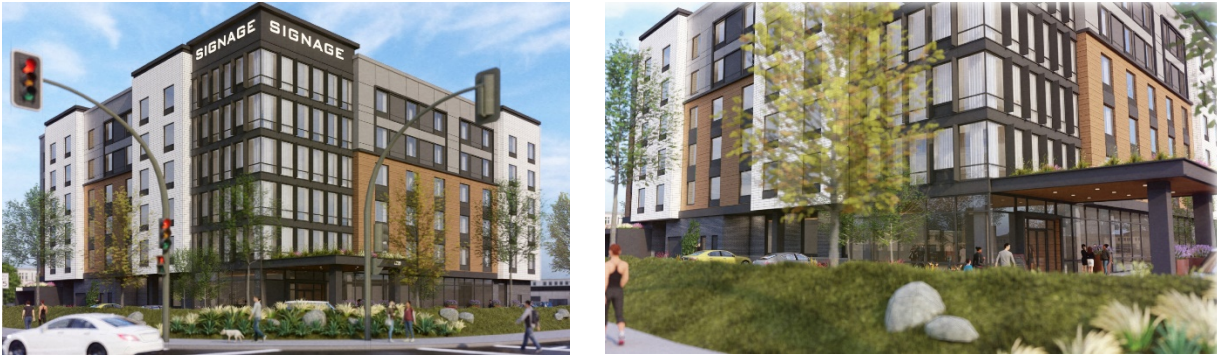
Figure 4. The building façades incorporate extensive opaque wall panels, mullions, awnings, and vertical metal fins, which help birds perceive the building as a solid structure (rather than as reflected sky or vegetation).
