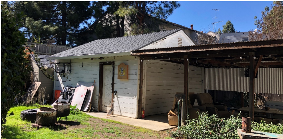
Figure 4. The detached garage behind 148 Crescent Avenue.
