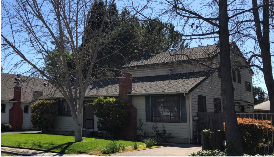
Figure 2. The front (north) and west façades of 148 Crescent Avenue.
