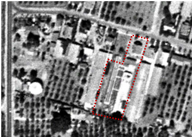
1948 aerial photograph of the area, the subject parcel outlined by the dashed red line (Google Earth).
