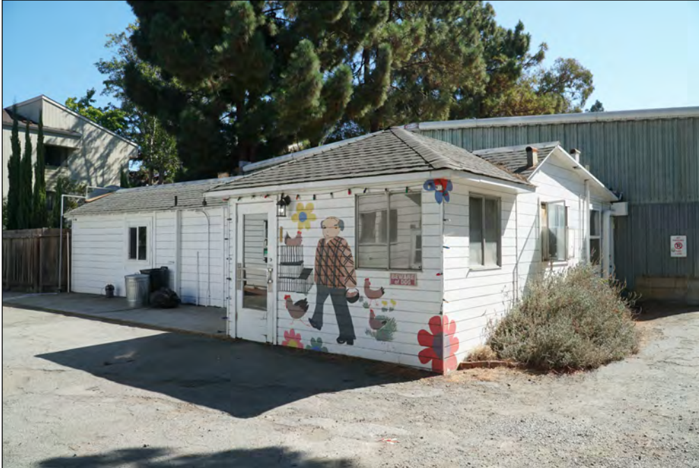
Figure 2. Looking southeast at north and west sides of office, 9/16/21.
