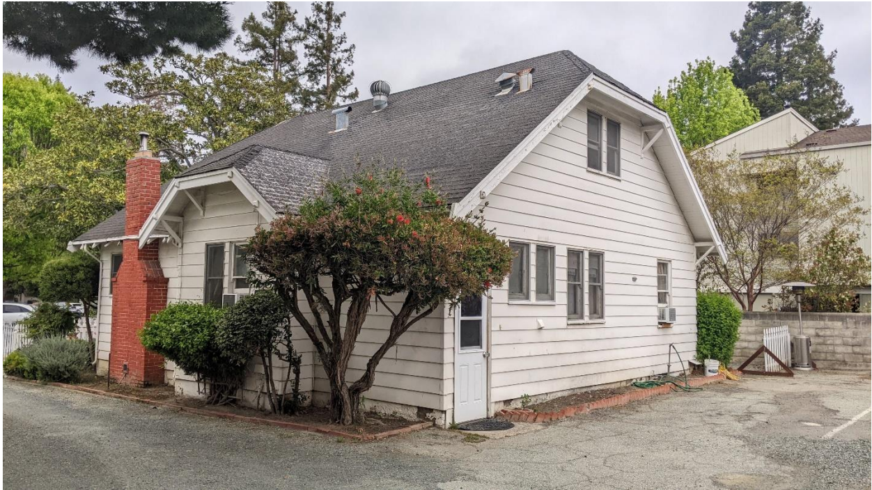
Figure 10. Rear, south facade of 156 Crescent Avenue, view northeast.
