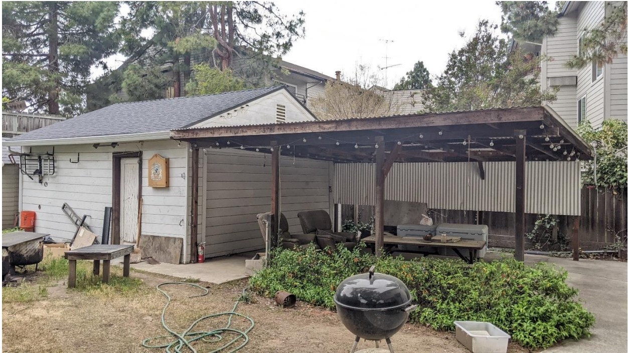
Figure 6. The garage and wood awning, view southwest.
