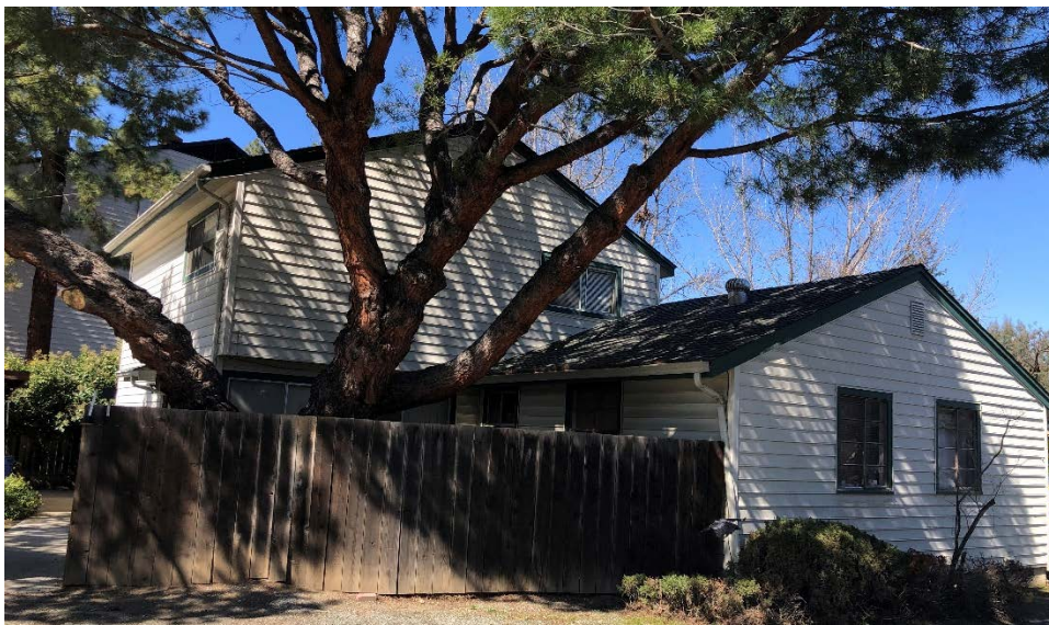
Figure 3. The east and south façades of 148 Crescent Avenue.
