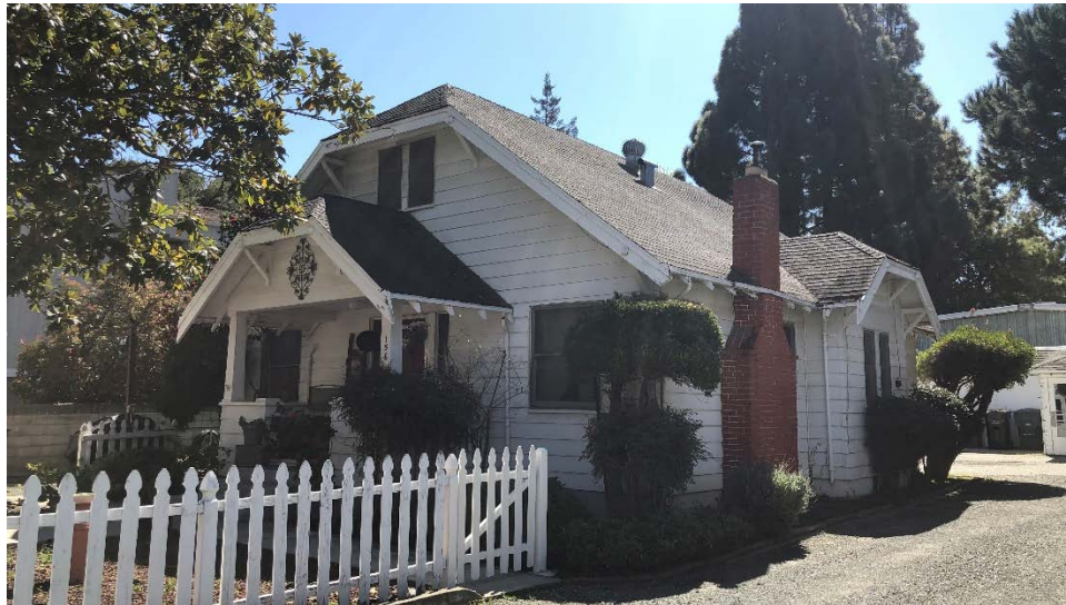
Figure 5. The front (north) and west façades of 156 Crescent Avenue.
