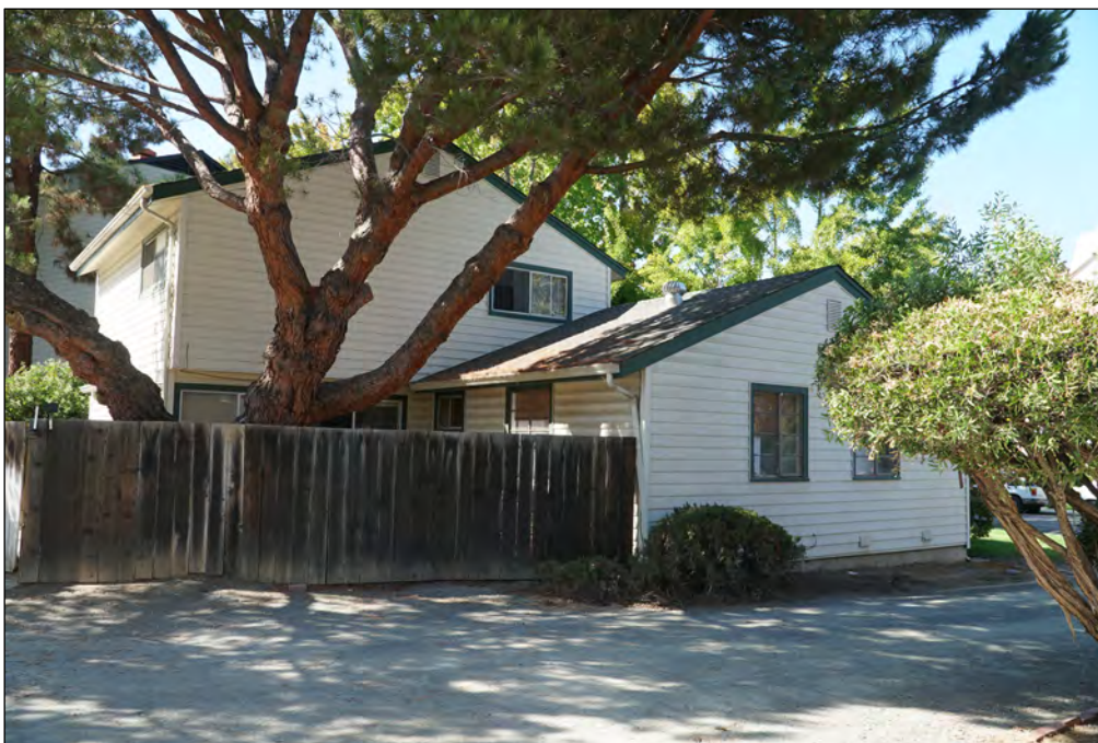
Figure 1. Looking northwest at south and east sides, 9/16/21.
