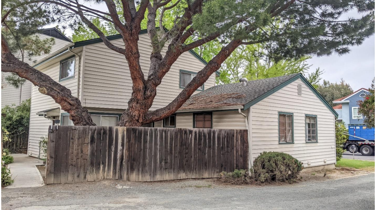
Figure 2. The east facade, view northwest.
