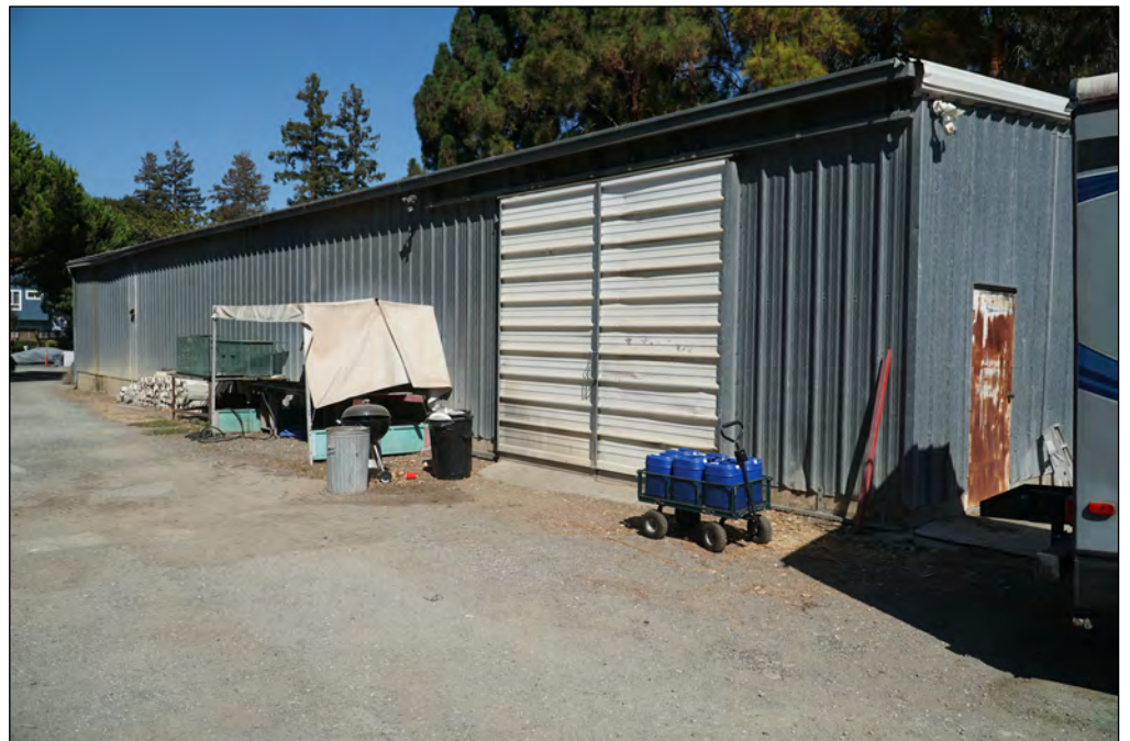
Figure 3. Looking northeast at west and south sides of warehouse, 9/16/21.
