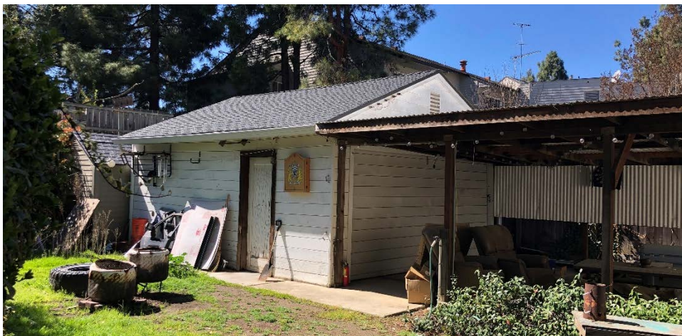
Figure 4. The detached garage behind 148 Crescent Avenue.
