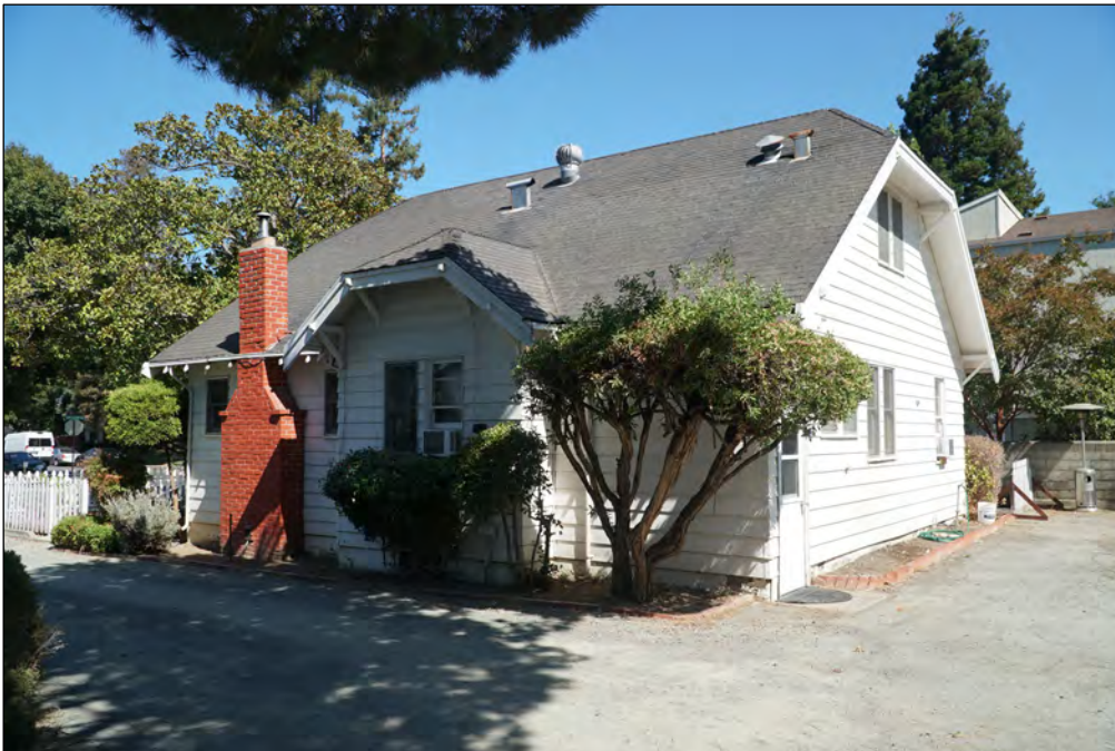
Figure 1. Looking northeast at west and south sides, 9/16/21.
