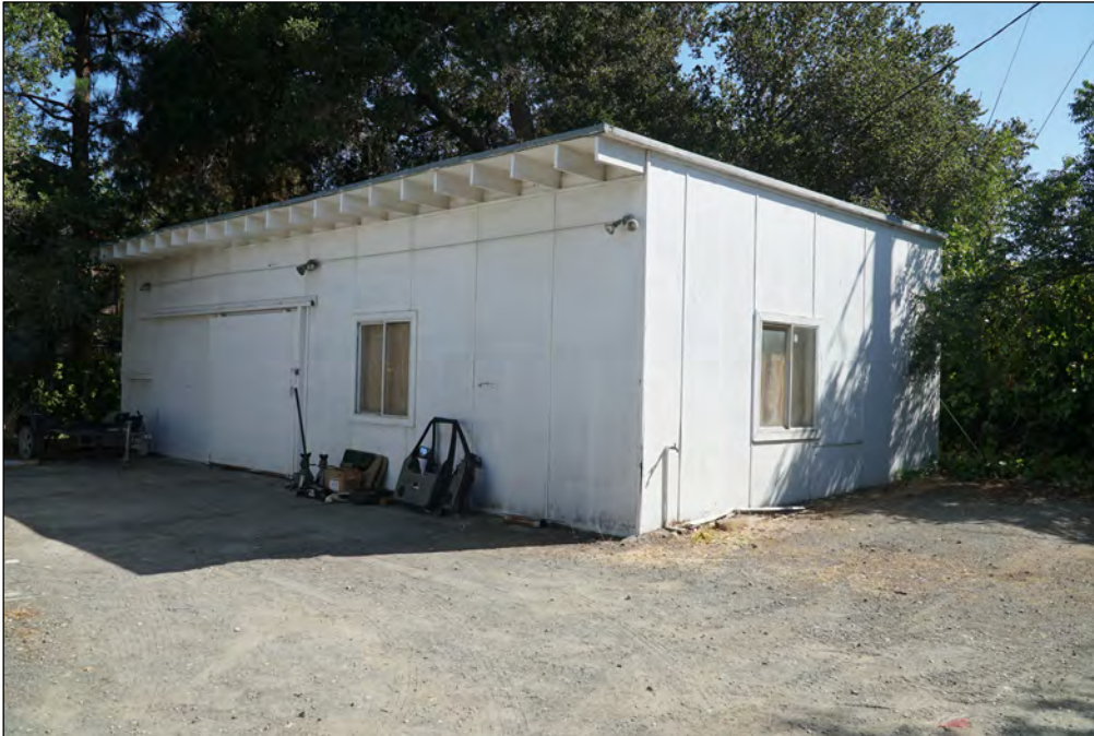
Figure 4. Looking south at north and west sides of shed, 9/16/21.
