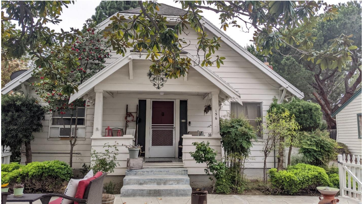
Figure 8. The primary, north façade of 156 Crescent Avenue, view south.
