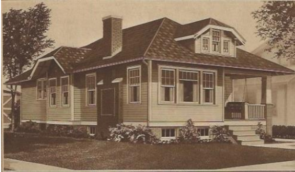
Figure 28. Craftsman-style kit house in the 1927 Sears, Roebuck and Co. Modern Homes catalog. Source: Sears, Roebuck and Co., Honor Bilt Modern Homes , 1927, Internet Archive.
