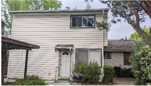
Figure 3. The south façade of the rear addition, view north.
