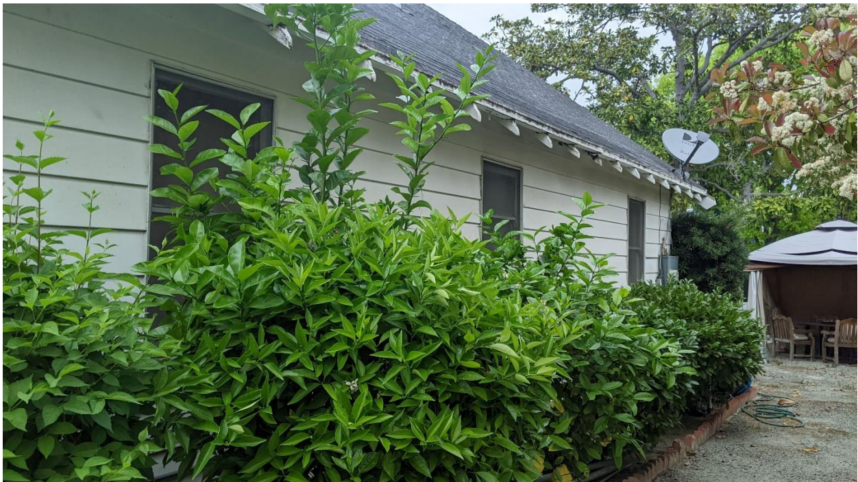
Figure 11. East façade of 156 Crescent Avenue, view south.
