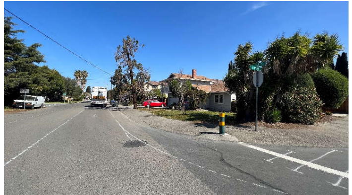
Bryant Way Intersection, North
