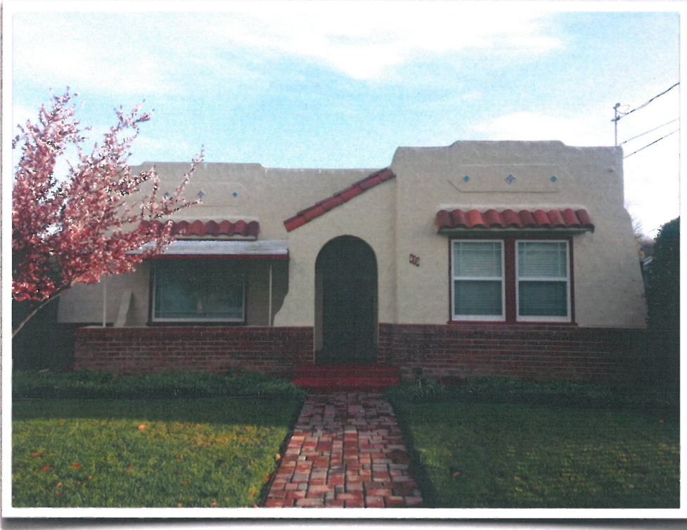
Front View – Mediterranean style stucco, flat roof, ceramic tile, and styling with blue and white tile
