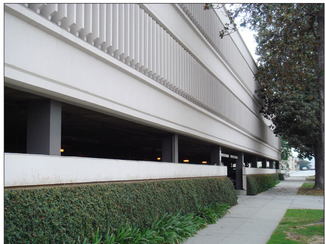
Cast-in-place concrete incorporating precast concrete elements
