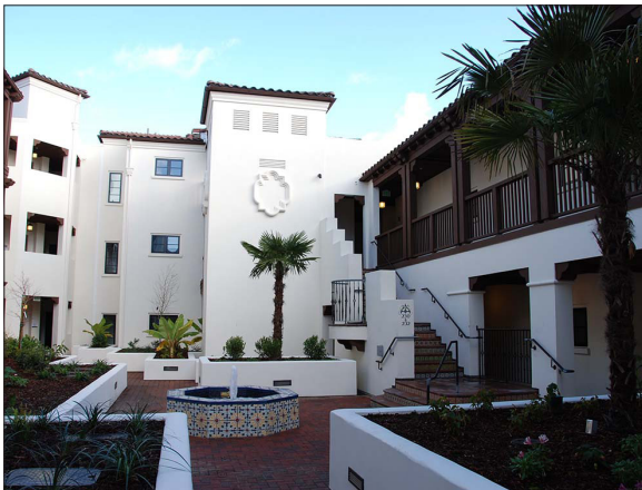
Landscaping on garage top with tall planters is not desirable
