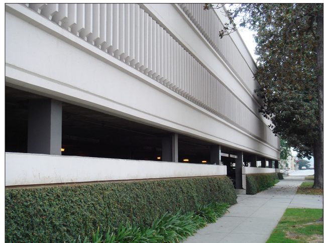
Cast-in-place concrete incorporating precast concrete elements
